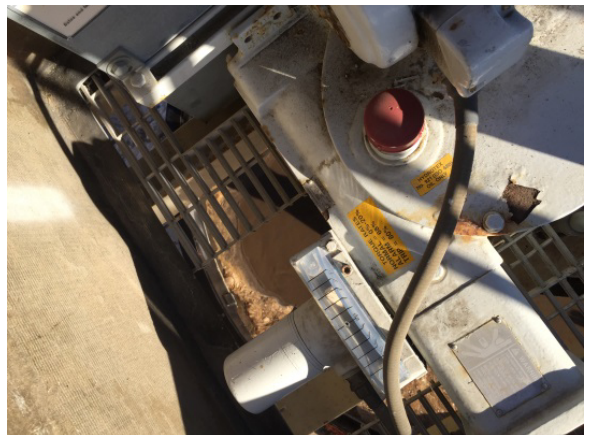
Minor Rust on Secondary Clarifier Drive, localized at coating breach
