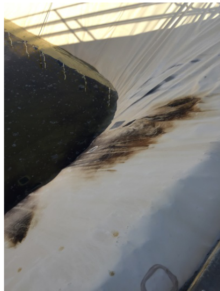
Equalization basin liner wear and discoloration
