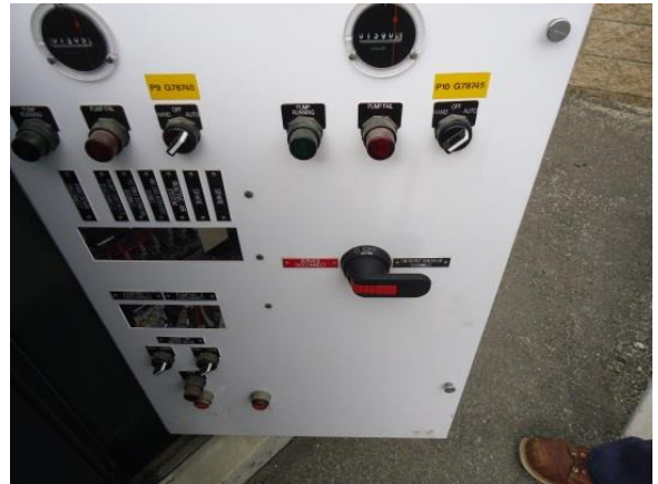
Control panel inner door with operators
