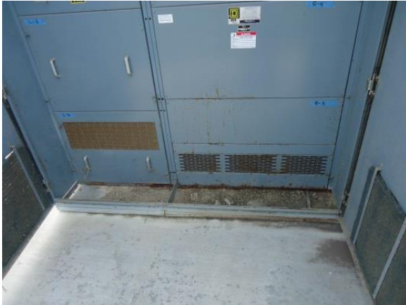
Outside switchboard corrosion from water ingress
