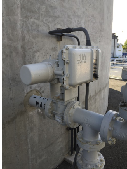
Mechanical piping and electric actuator
