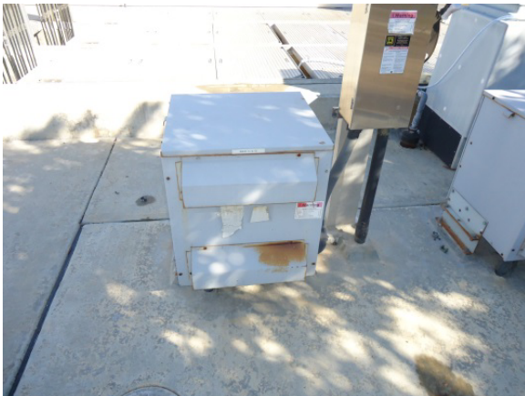
Rust on UV transformer
