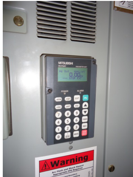
Mitsubishi VFD operator keypad
