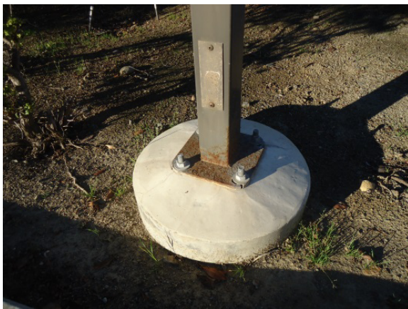
Rust on base of site lighting pole
