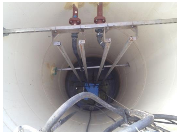
Cerro Del Sol #1 wet well in excellent condition
