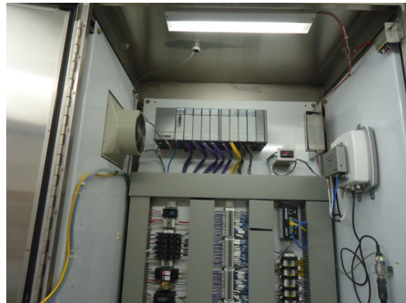
Remote site PLC control panel
