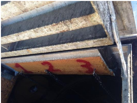
Corrosion on underside of wet well hatch
