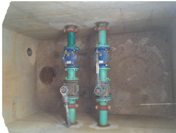
Valve Vault Piping, Fittings, and Valves
