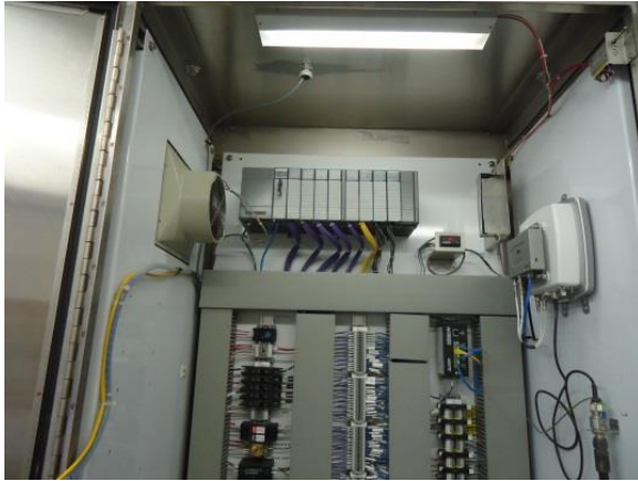
PLC panel with Cisco Aironet Ethernet radio
