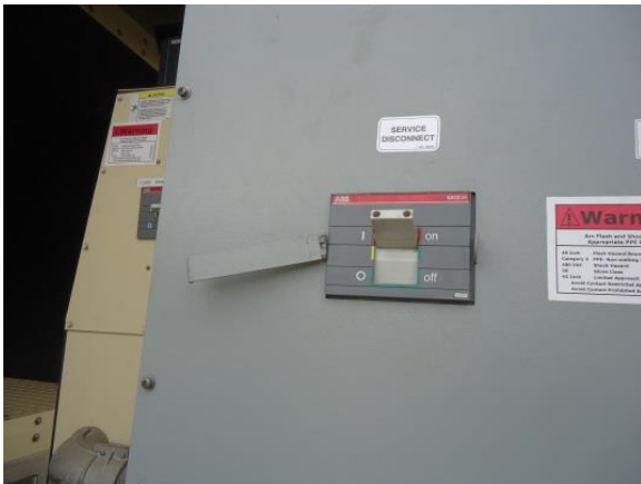
Generator main disconnect lockout (not working)
