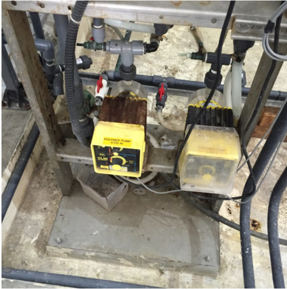
Minor corrosion on polymer skid and equipment
