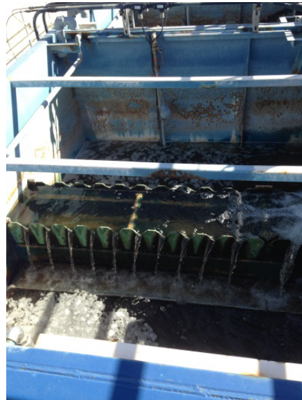
Filter bed corrosion and wear
