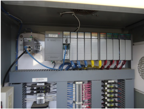
Blower PLC panel interior view
