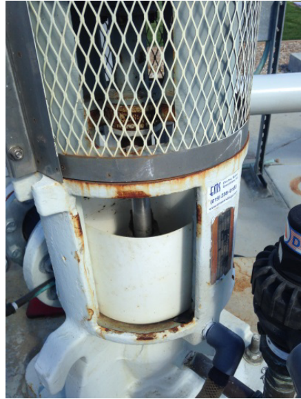
Minor rust on non-potable water pump
