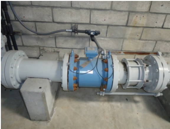
Rosemount Flowmeter Element
