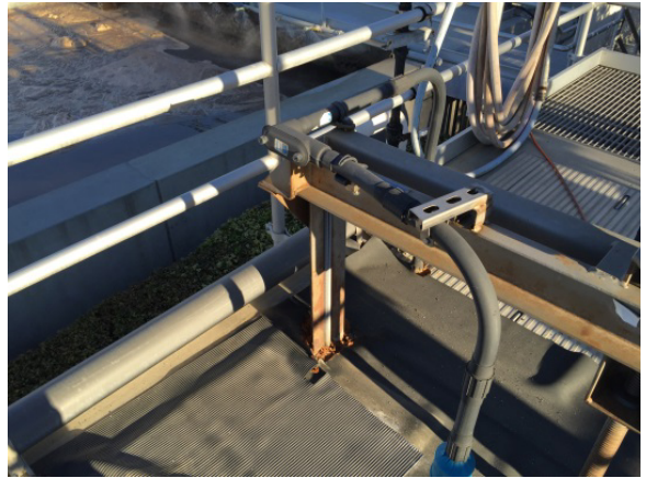
Rust on Steel gate frame
