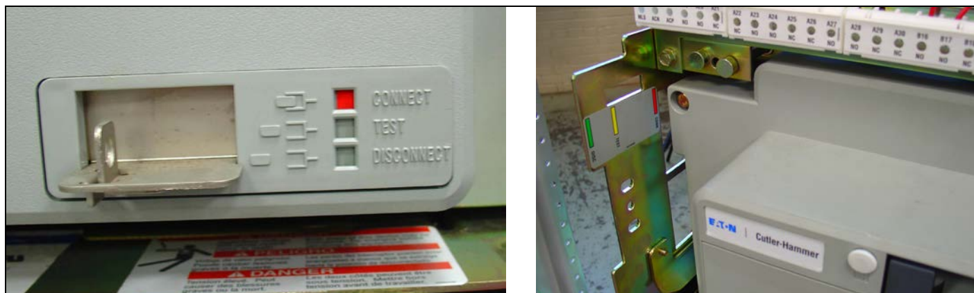
Figure 30. Switching Device in the CONNECT Position.
