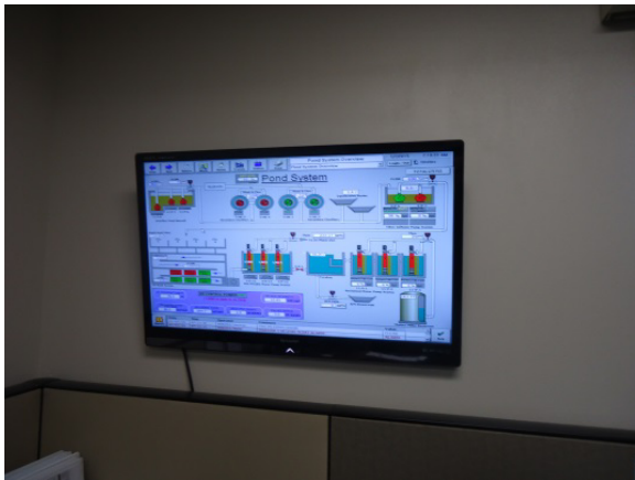
SCADA central HMI color screen
