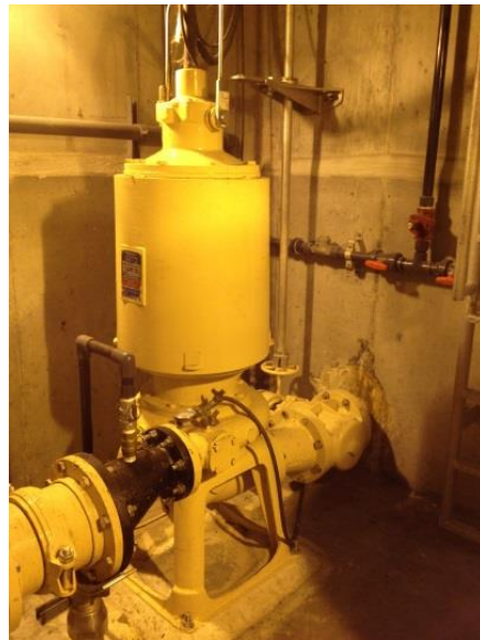
Fire House dry well submersible pump
