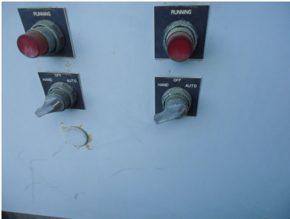
Outdoor local control panel pitted operators
