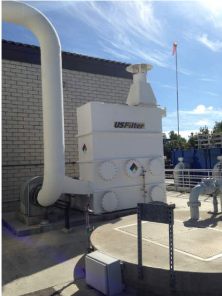
Sludge Dewatering Building odor control scrubber
