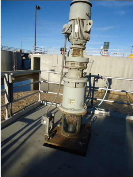
Corrosion on base of Anoxic Tank Mixer
