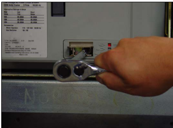
Figure 34. Levering and Position Indication.
