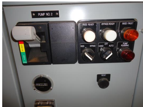
Pump 2 motor control bucket
