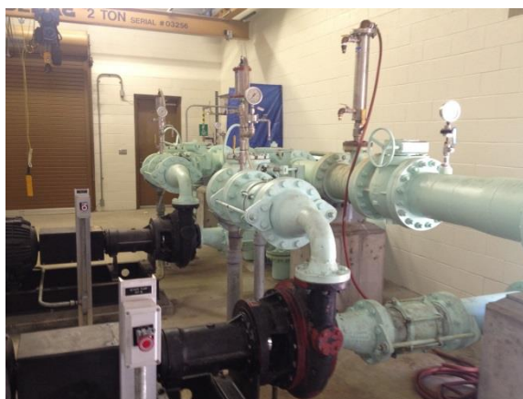
Del Dios pumps and mechanical piping
