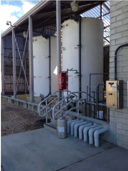
Recently replaced Sodium Hypochlorite Tanks
