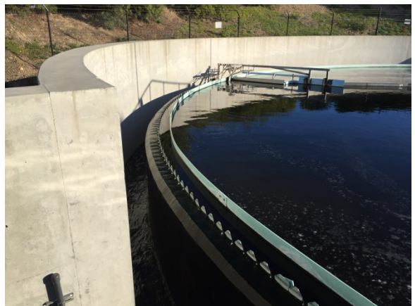
Clarifier structure and skimmer
