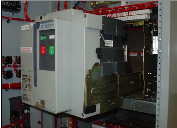
Figure 27. Switching Device Drawn Out from the Transfer Switch.
