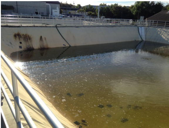
Equalization basin liner wear and discoloration
