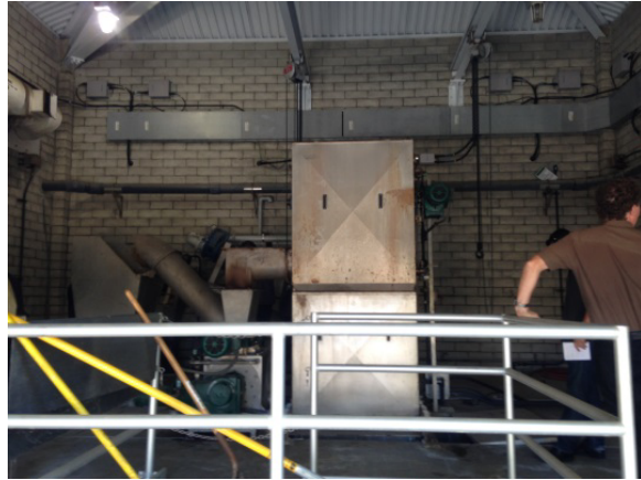
Corrosion on Bandscreen
