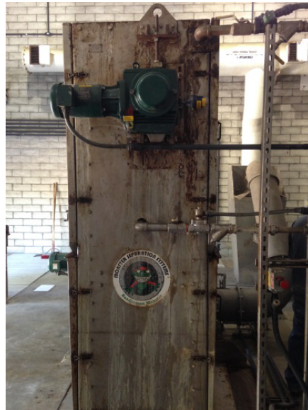
Corrosion on Bandscreen
