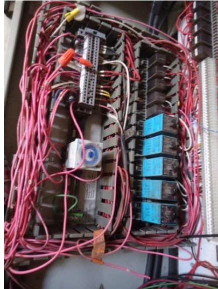
VFD control section wire mess
