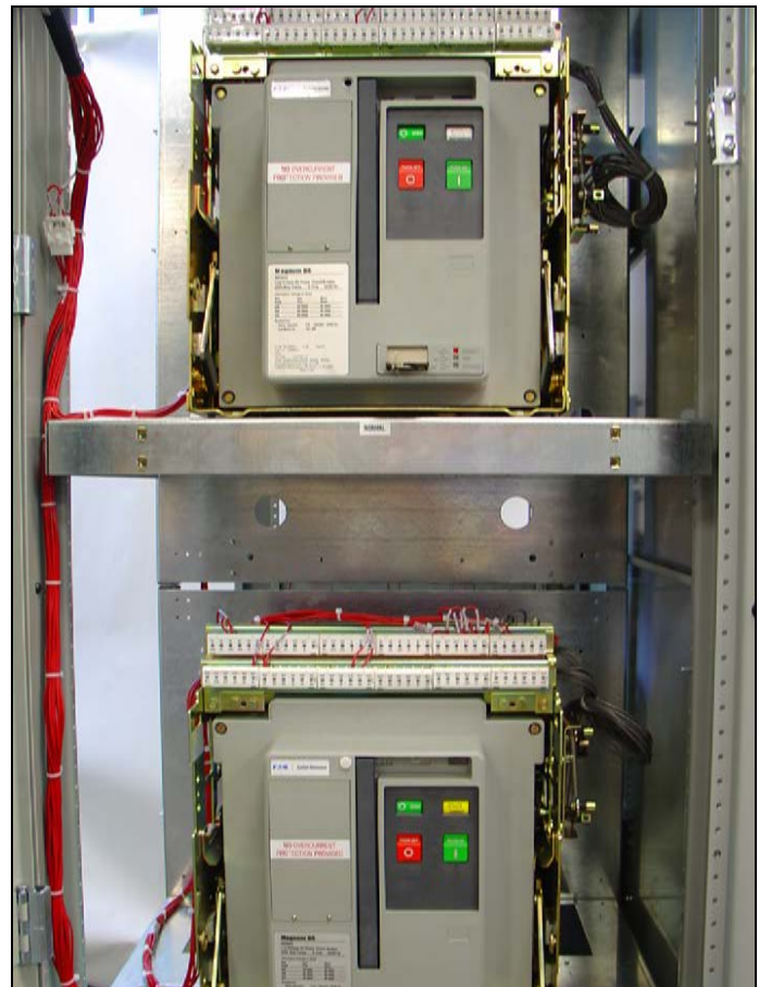
Figure 11. Typical Power Compartments (Open Transition Shown).
