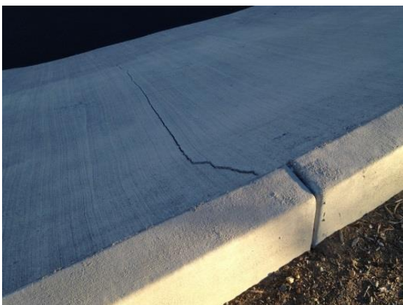
Cracking observed in emergency storage pond
