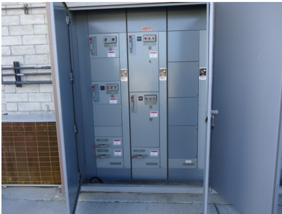
MCC installed outside of electrical room
