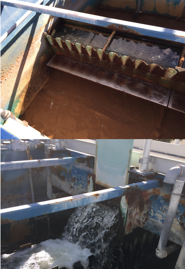
Figure 4: Filter Corrosion Damage
