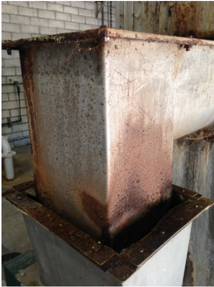
Corrosion on chute from screen to grinder, wash/press
