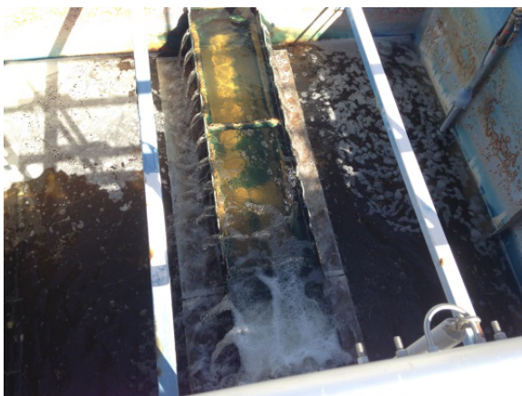
Filter bed corrosion and wear
