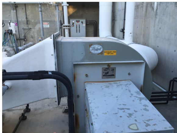
Minor corrosion on headworks odor control fan
