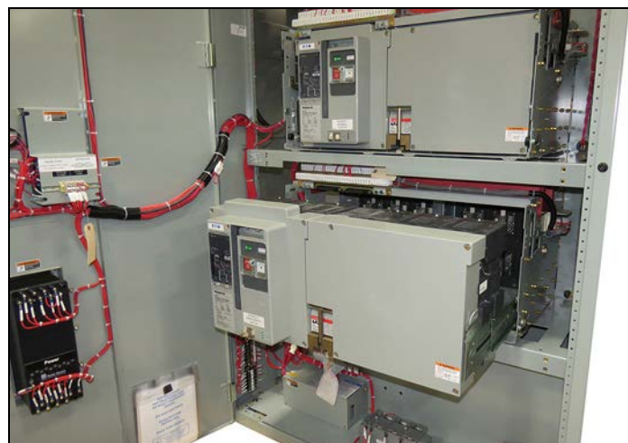
Figure 9. Drawout Switching Device Fully Extended from the Magnum Transfer Switch.
