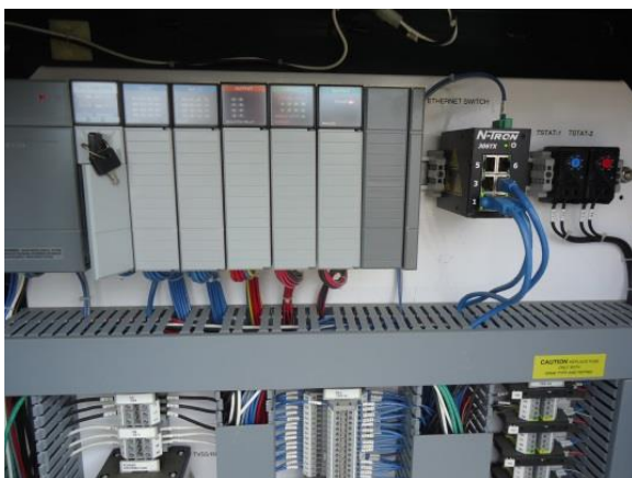
Control panel PLC section
