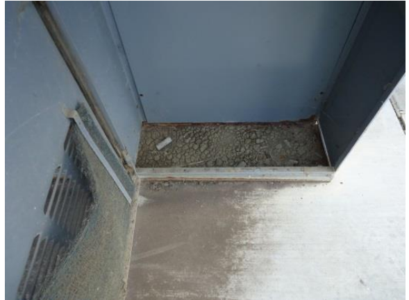
Outside switchboard corrosion from water ingress
