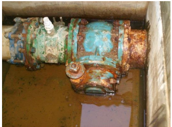
Rust and corrosion on mechanical piping and isolation valve
