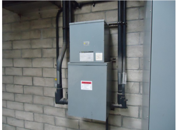
Mini power station, combo transformer and panelboard
