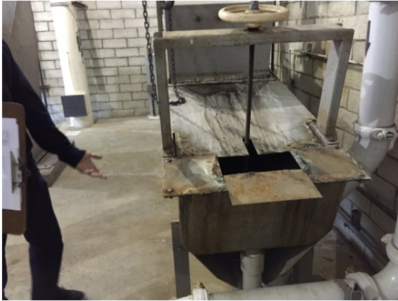
Corrosion on Grit Classifier
