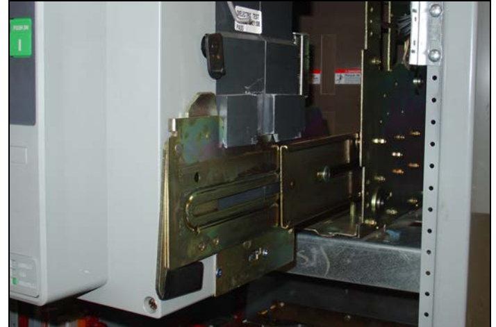
Figure 29. Switching Device in the REMOVE Position.
