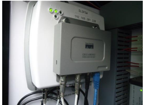
Cisco Aironet Ethernet radio
