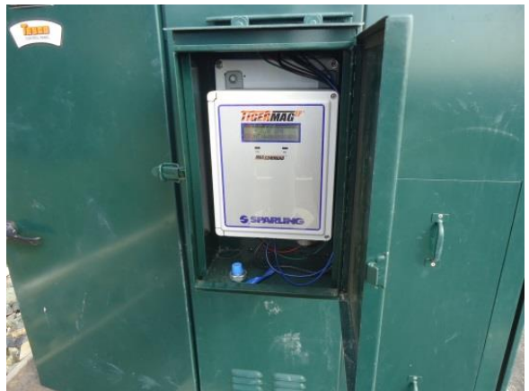
Flow transmitter mounted in control panel side-mounted enclosure
