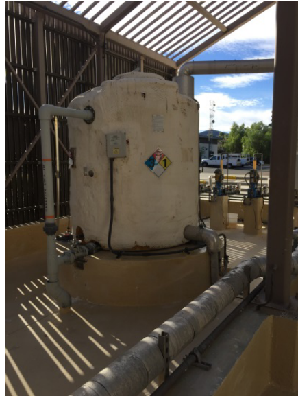
Insulation deterioration on caustic soda storage tank
