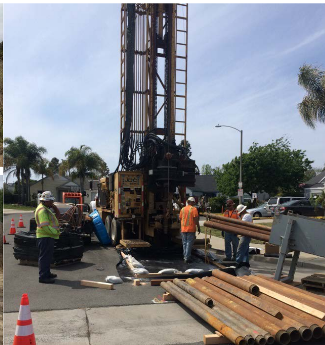
Photo 2: Example Test Well during Construction
