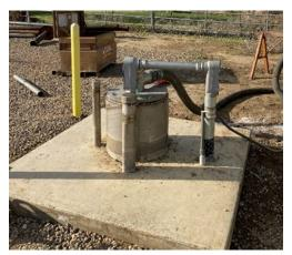
Figure 3-1. Wellhead completed 24-inches above 100-year flood plain.
