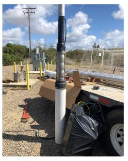
Figure 7-1. Permanent pump prior to installation.
