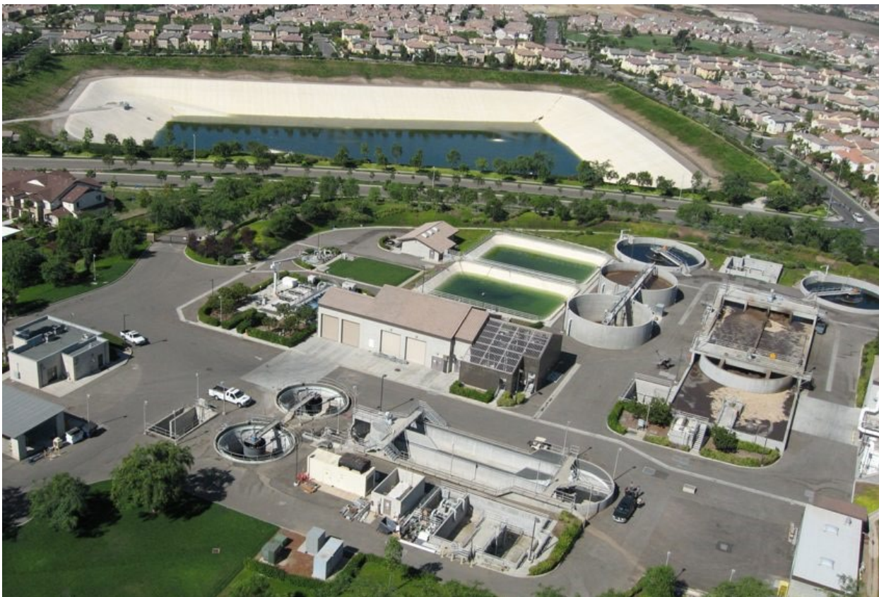
4S Reclamation Facility and Recycled Water Pond
