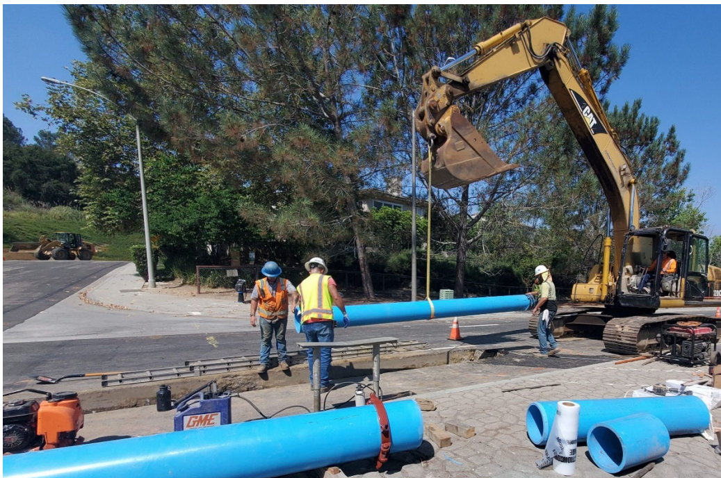
Construction crews installing the Unit A potable water pipeline
