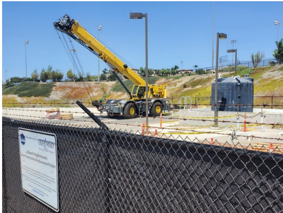
Replacement Neighborhood 1 Sewer Pump Station under construction.
