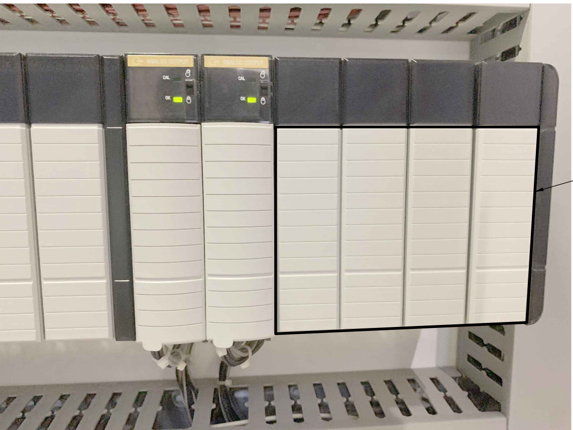
EXISTING PANEL CC-RHB PLC RACK 26 (REMOTE I/O) SPARE SLOTS
