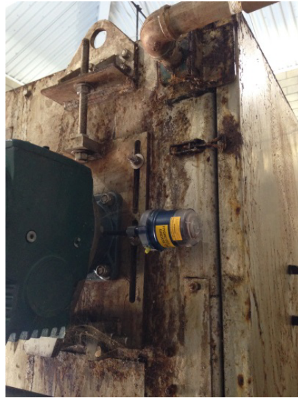
Corrosion on Bandscreen and fittings
