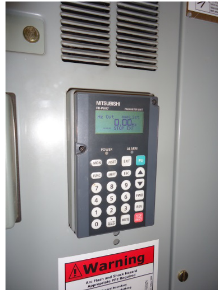
Mitsubishi VFD operator keypad
