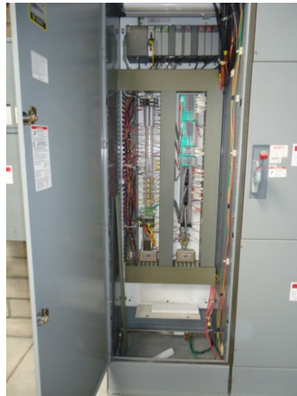
PLC-3 control panel interior view
