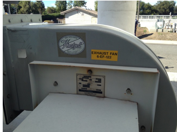
Sludge Dewatering Building odor control fan
