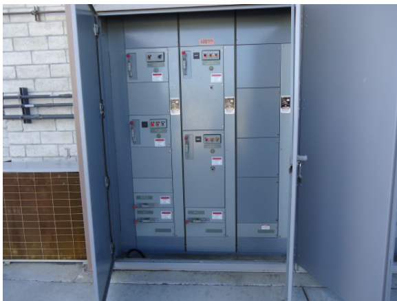
MCC installed outside of electrical room
