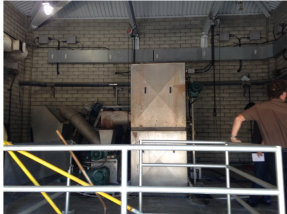
Corrosion on Bandscreen
