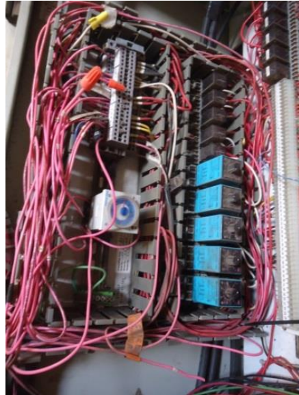
VFD control section wire mess
