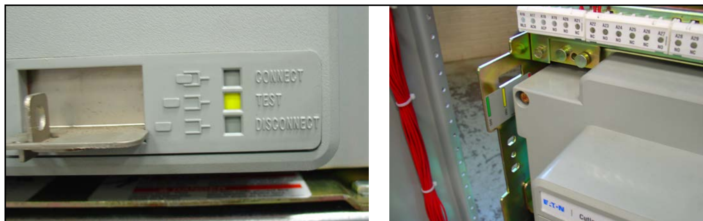
Figure 31. Switching Device in the TEST Position.
