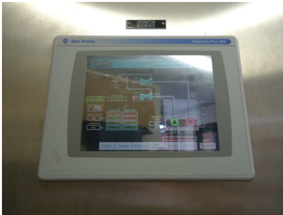
Remote site operator interface terminal (OIT)
