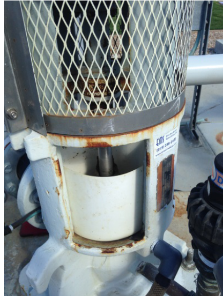
Minor rust on non-potable water pump
