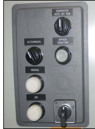
Figure 36. Typical Bypass Isolation Transfer Switch Device Panel.
