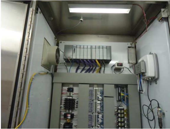
PLC panel with Cisco Aironet Ethernet radio
