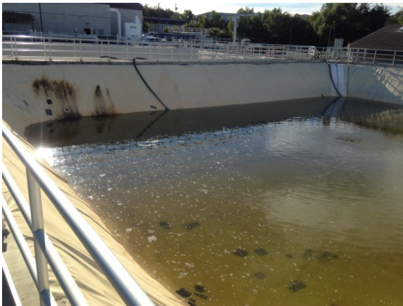
Equalization basin liner wear and discoloration
