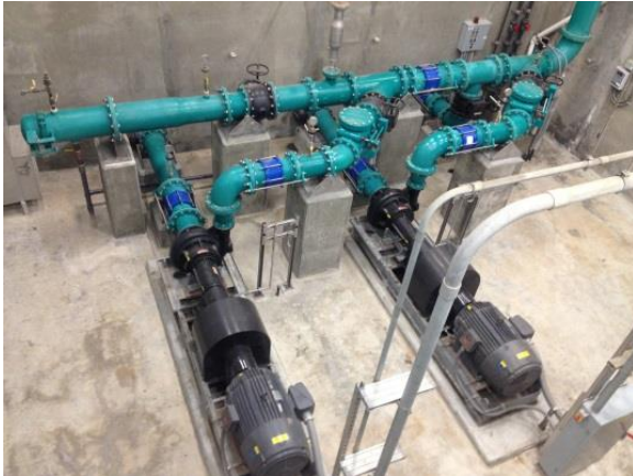
Neighborhood #3 pumps, motors, and mechanical piping (from above)
