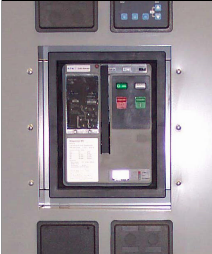
Figure 12. Power Case Switching Device.
