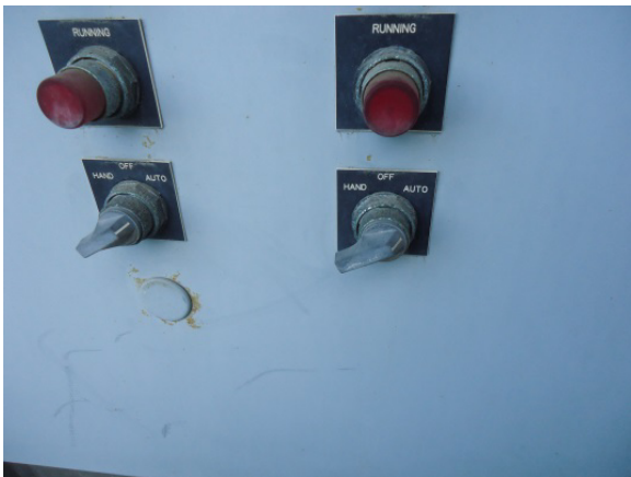
Outdoor local control panel pitted operators
