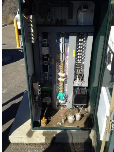
Water accumulated inside base of control panel
