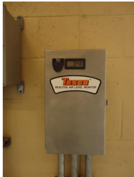
Tesco reactive air level system
