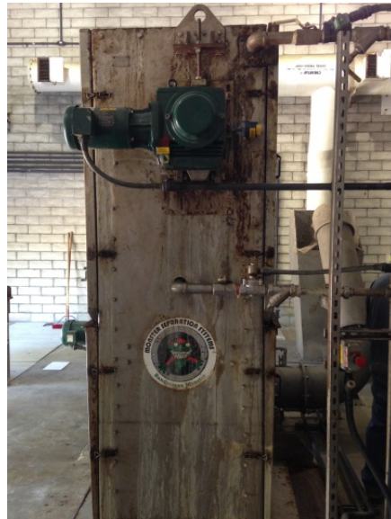
Corrosion on Bandscreen
