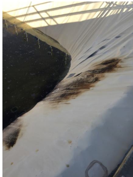
Equalization basin liner wear and discoloration
