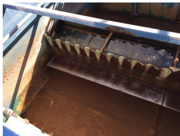
Filter bed corrosion and wear
