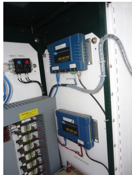
Dual iNet Ethernet radios
