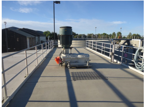
Oxidation Ditch Aerator
