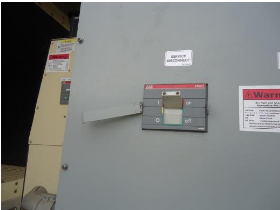
Generator main disconnect lockout (not working)
