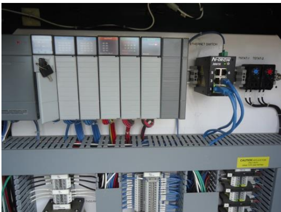
Control panel PLC section
