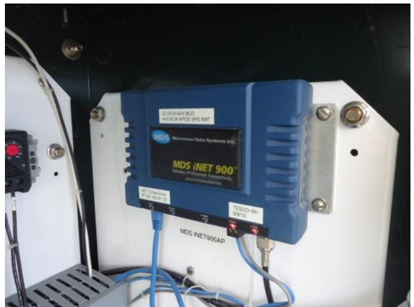
MDS iNet Ethernet radio
