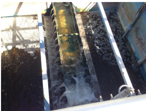
Filter bed corrosion and wear
