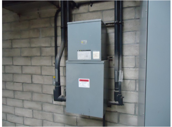
Mini power station, combo transformer and panelboard
