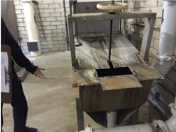
Corrosion on Grit Classifier
