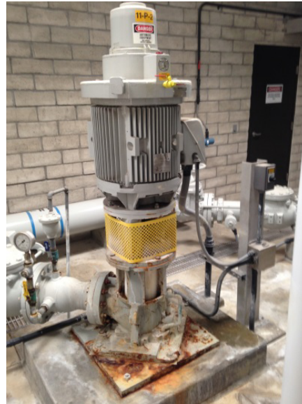
Minor Rust on baseplate of recycled water pump
