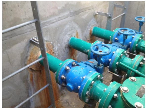
Concrete corrosion around valve vault pipe penetration
