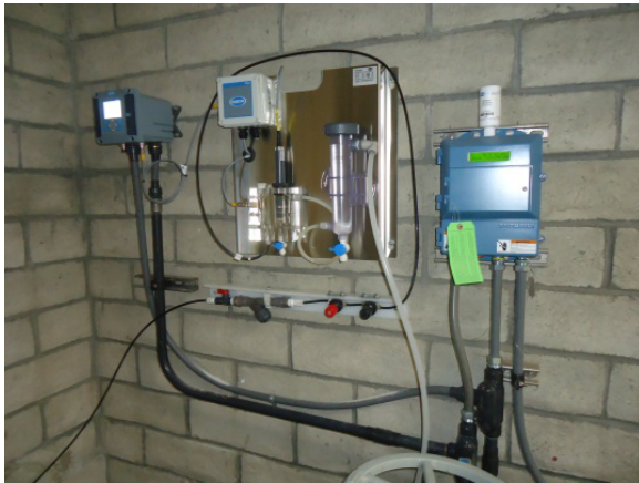
Pump station water quality analyzers
