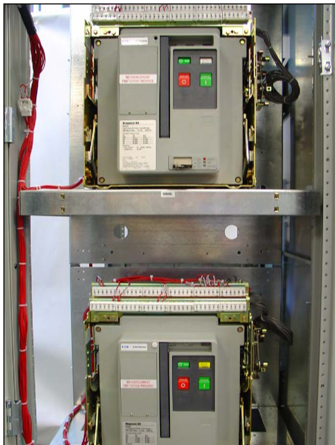
Figure 11. Typical Power Compartments (Open Transition Shown).
