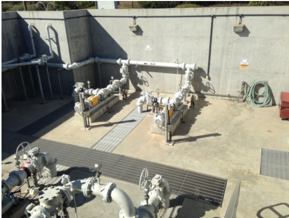
RAS/WAS pump station structure
