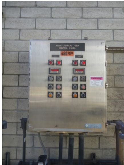
NEMA 4X SS chemical metering pump control panel
