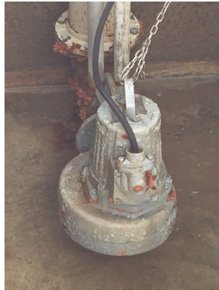
Corrosion of anode and bubbling/cracking of filter backwash pump coating
