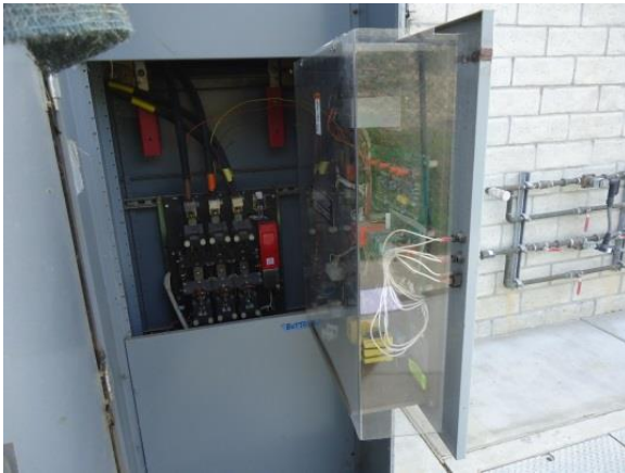
Outside switchboard ATS section
