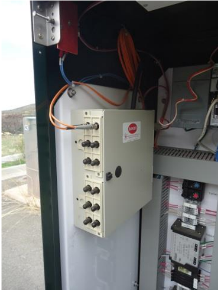
Fiber optic termination closet
