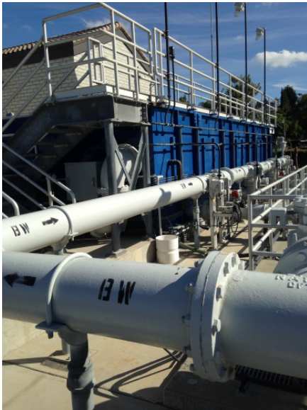
Tertiary Filters and mechanical piping
