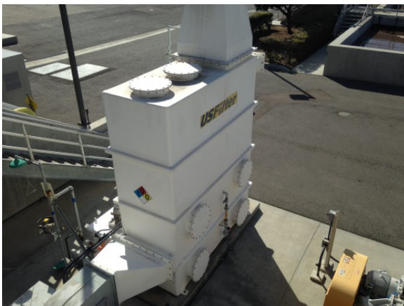
Headworks Odor Control Scrubber
