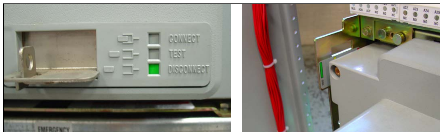
Figure 32. Switching Device in the DISCONNECT Position.
