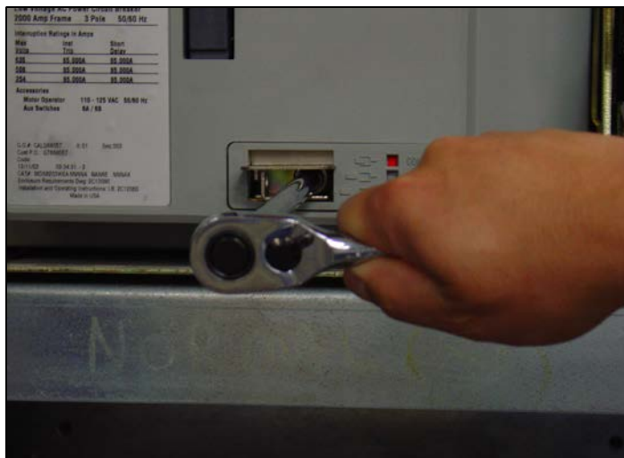
Figure 34. Levering and Position Indication.
