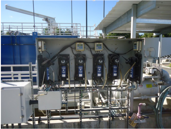
Filter turbidity analyzers
