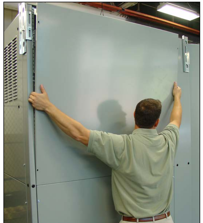
Figure 42. Lifting the Cover Free.
