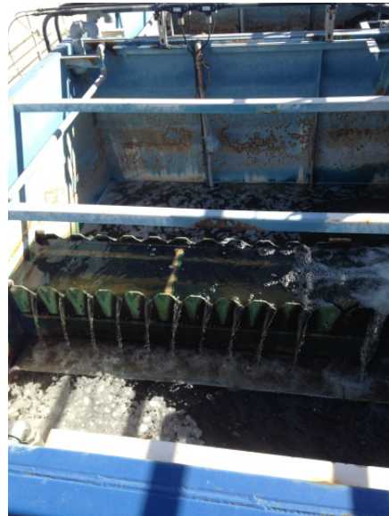
Filter bed corrosion and wear
