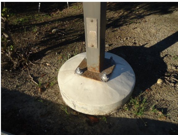
Rust on base of site lighting pole
