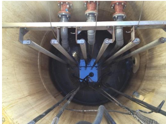
Cerro Del Sol wet well in excellent condition
