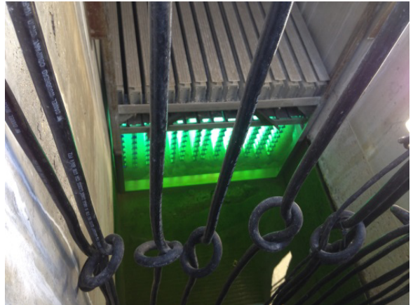
On-line UV bank in channel
