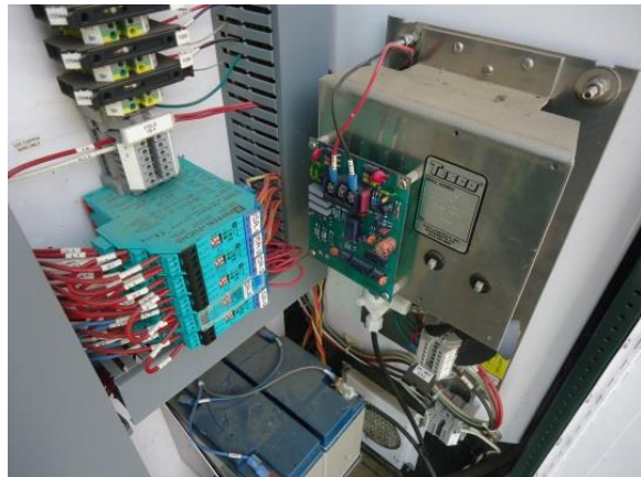
PLC section with Tesco reactive air level system
