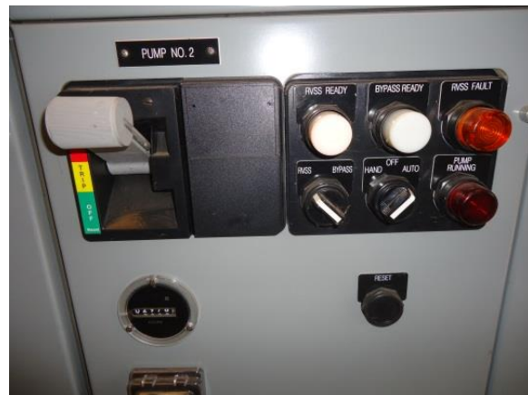
Pump 2 motor control bucket
