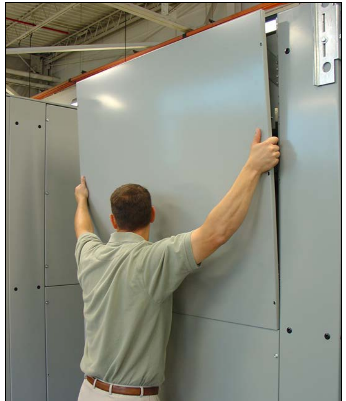
Figure 41. Tilting the Cover Away from the Frame.
