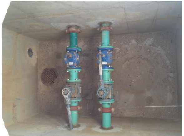
Valve Vault Piping, Fittings, and Valves
