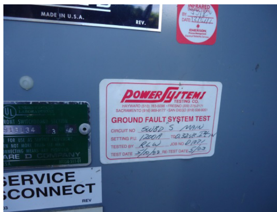
Service disconnect outdated electrical testing sticker
