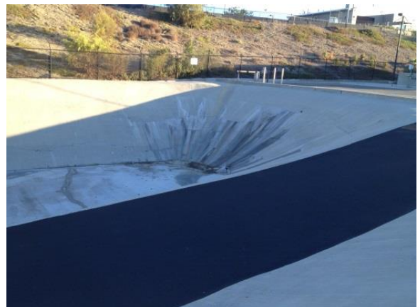
Groundwater intrusion and discoloration observed in emergency storage pond
