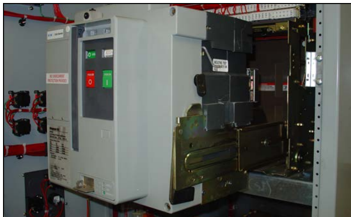
Figure 14. Drawout Mechanism (Closed Transition Shown)
