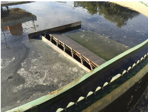
Minor Rust on Secondary Clarifier Mechanical and Weirs
