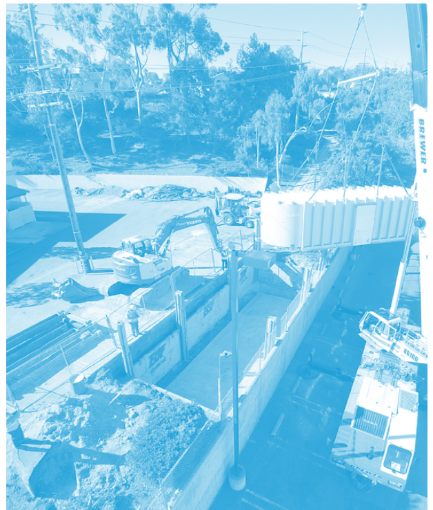
OMWD's Village Park Recycled Water Project included a reservoir conversion and the installation of a pump station and seven miles of pipeline in order to serve up to 114 million gallons of recycled water each year in Encinitas.
