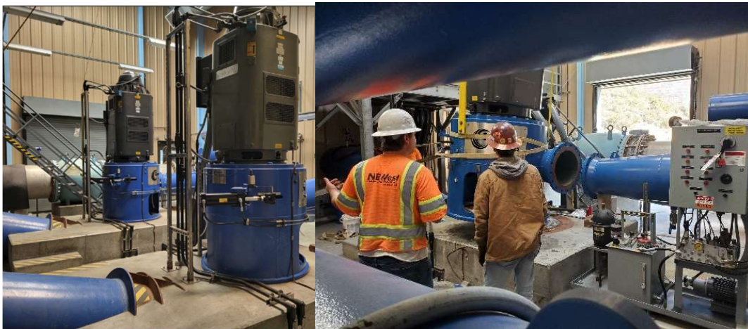
Refurbished turbines being reinstalled at the District's David C. McCollom Water Treatment Plant
