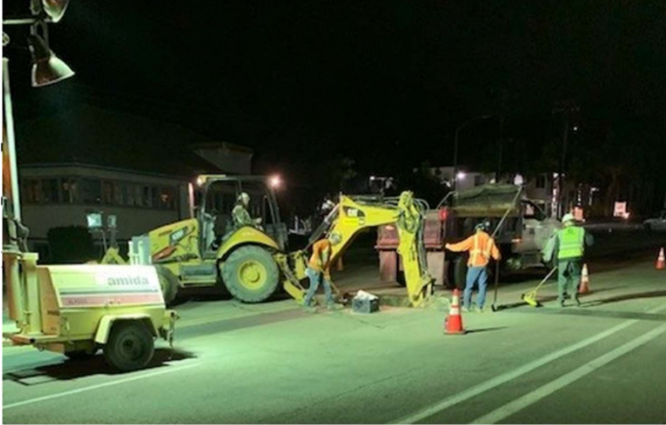
Night crew working to install new potable water pipeline along Manchester Avenue
