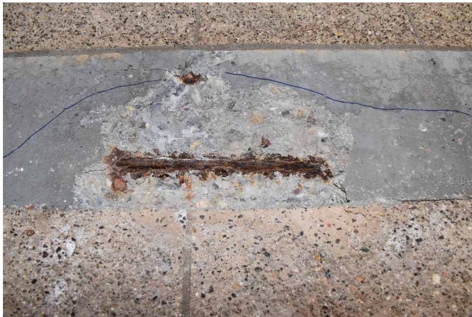
Photograph 26: Exposed Reinforcement in Thickened Slab Edge (03/22/2022)
