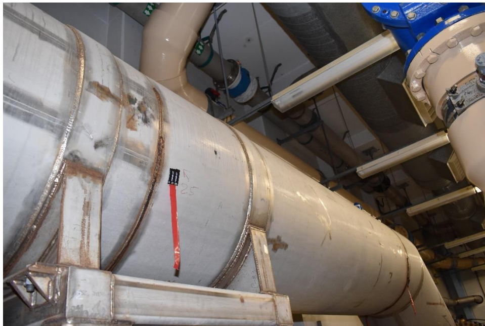
Photograph 28: Corrosion on Blower Room Piping (01/26/2022)
