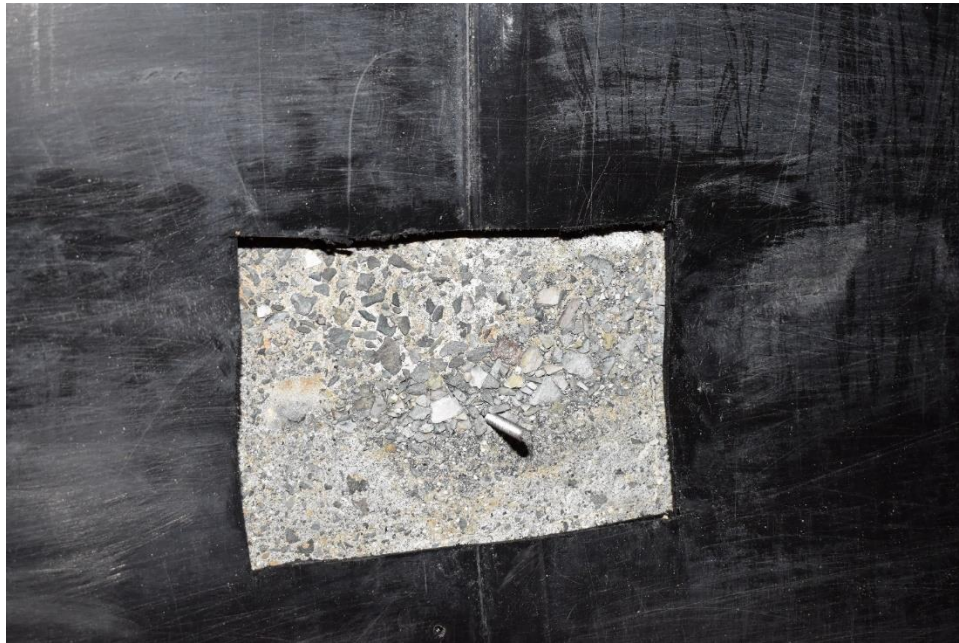
Photograph 5: Concrete at Lower Liner Cut on West Wall (01/26/2022)
