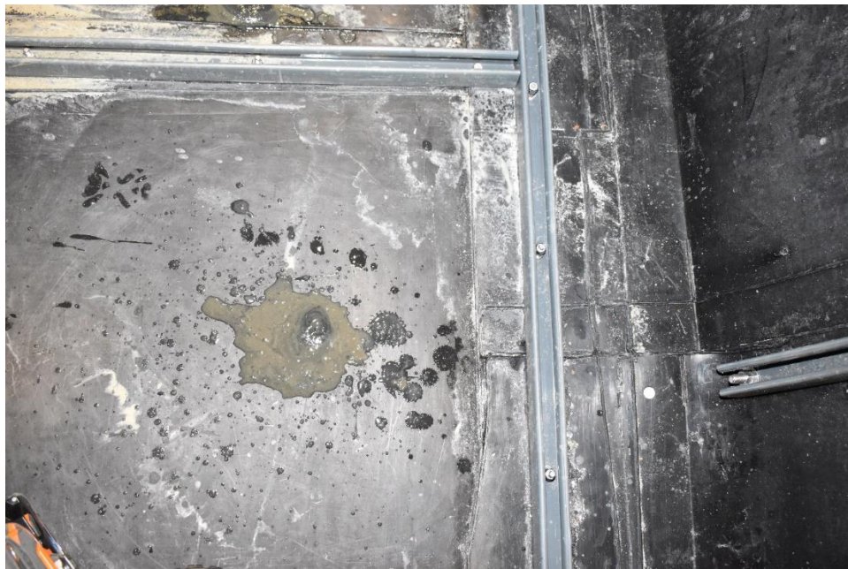
Photograph 6: Hole in Floor Liner and Sludge (01/26/2022)
