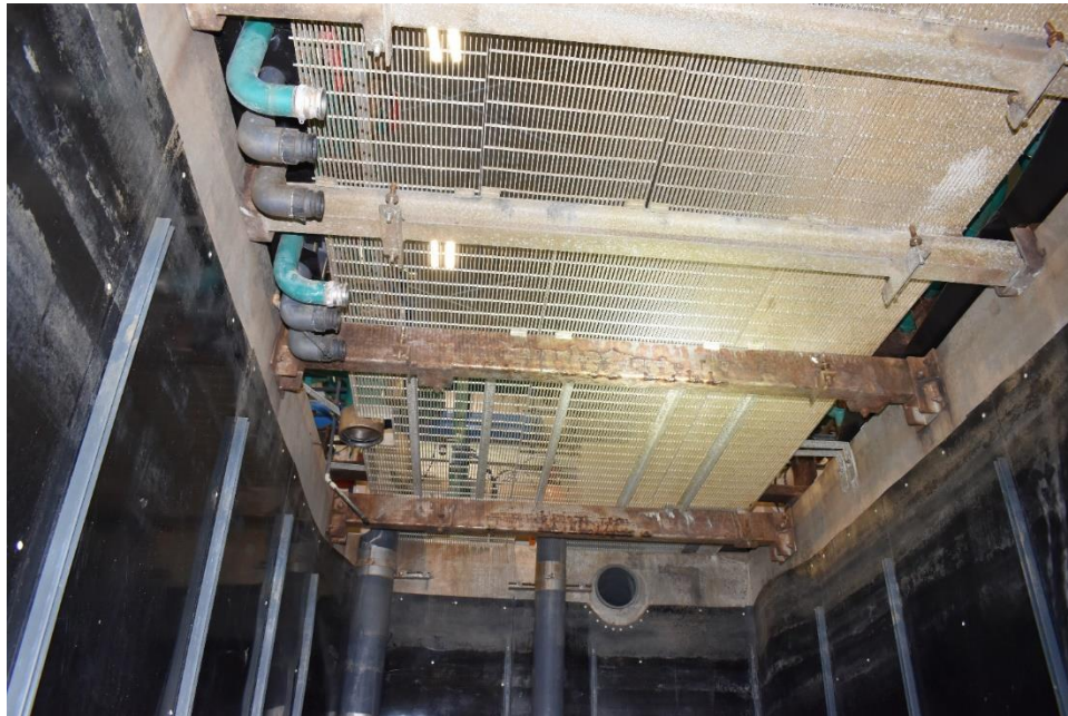
Photograph 7: Corrosion on Basin Steel Beams (01/26/2022)
