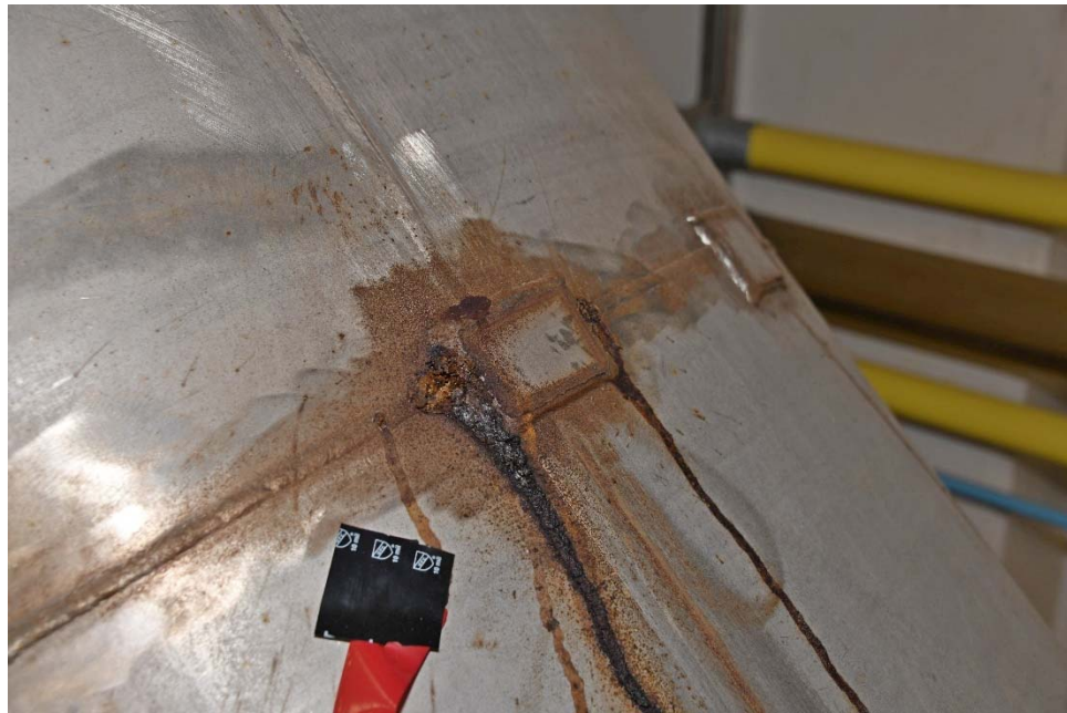
I-18 View of the topside of the pipe, illustrating a welded patch that appears to have been leaking.
