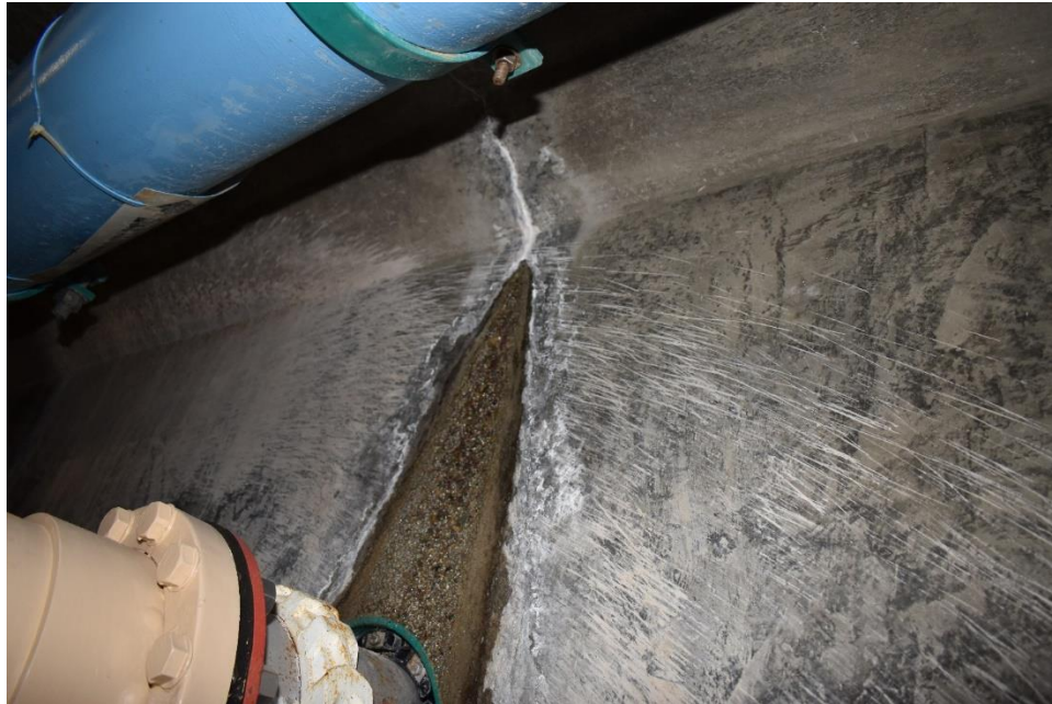
Photograph 9: Leaking Crack in Primary Stage Basin No. 3 (01/26/2022)
