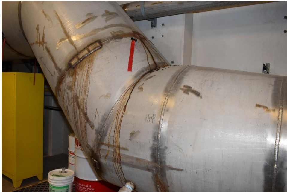
Photograph 27: Corrosion on Blower Room Piping (01/26/2022)
