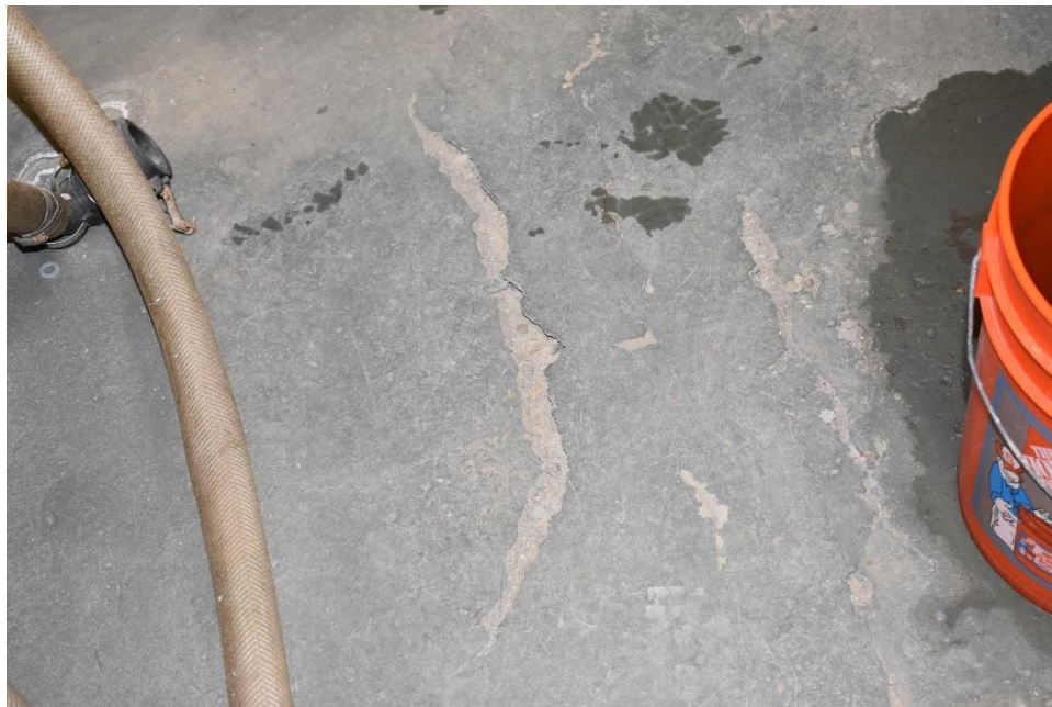
Photograph 12: Damage to Sodium Hypochlorite Room Floor Slab (01/26/2022)
