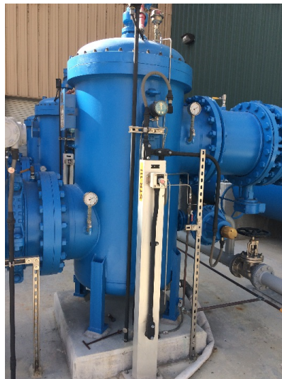
Figure 1-1. Bollfilter type 6.18/500 DN 500 Automatic Backwash Strainer
