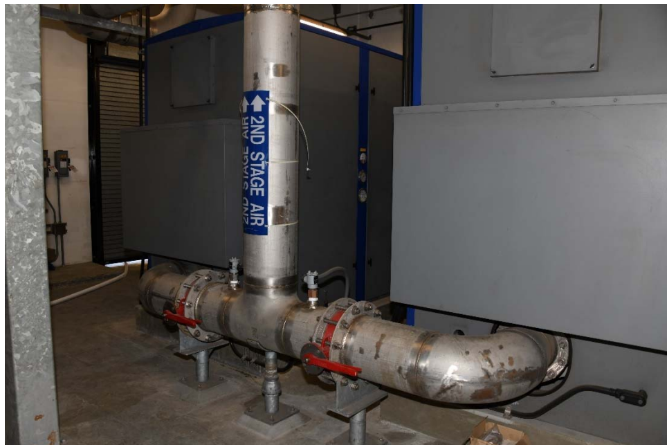
I-28 View of 2 nd stage air piping, illustrating very minor corrosion on the piping and along random welds.
