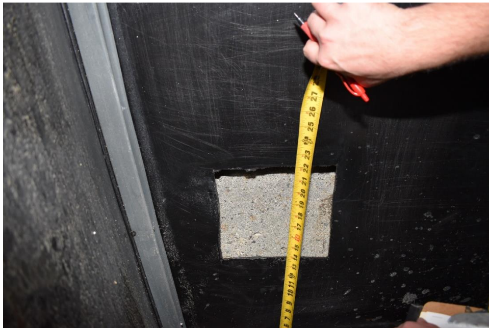
Photograph 4: Concrete at Lower Liner Cut on South Wall (01/26/2022)
