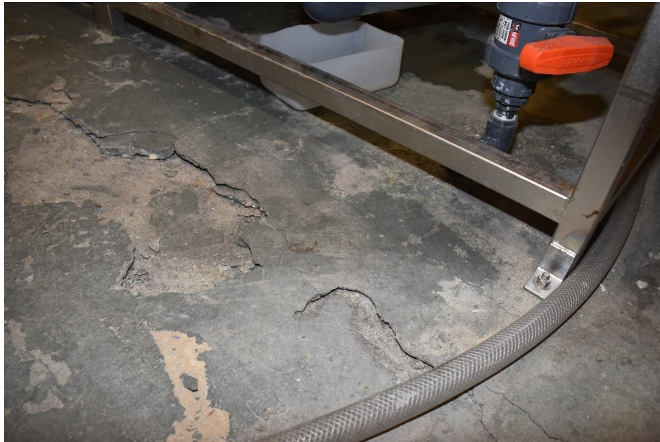
Photograph 11: Damage to Sodium Hypochlorite Room Floor Slab (01/26/2022)
