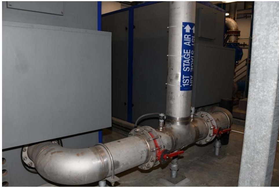
I-26 View of 1 st stage air piping, illustrating the overall good condition of the piping.
