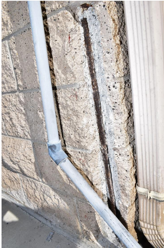
Photograph 22: Exposed Reinforcement at Southwest Corner of Fluoride Room (01/27/2022)
