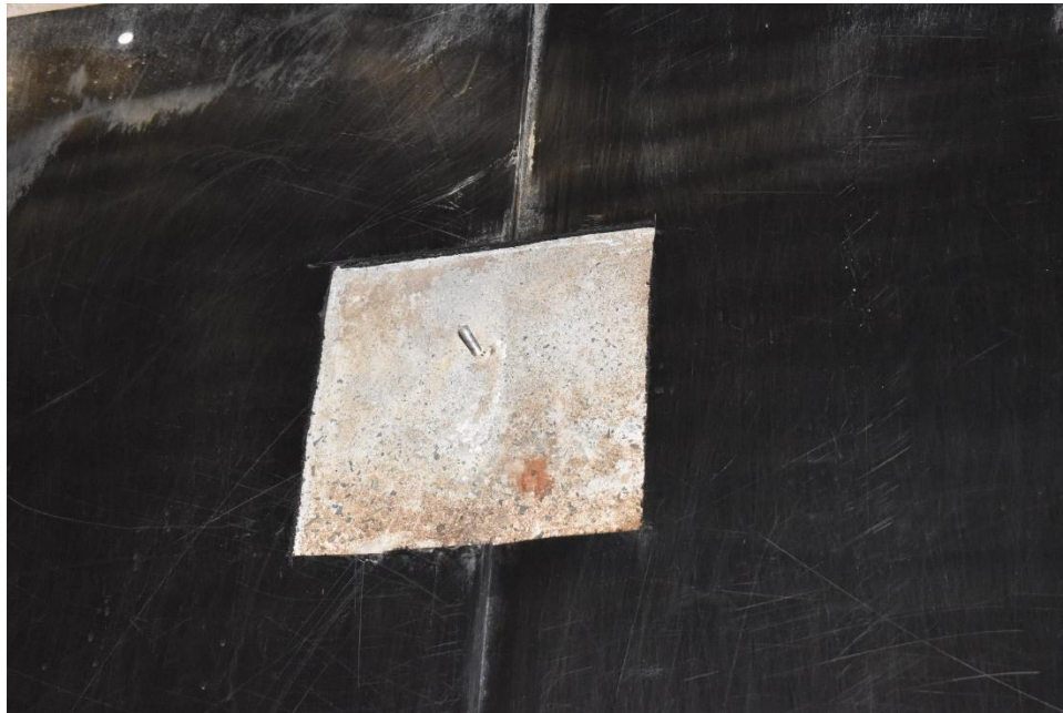
Photograph 3: Concrete at Upper Liner Cut on East Wall (01/26/2022)
