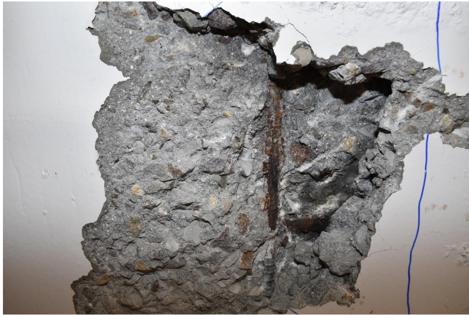
Photograph 23: Exposed Reinforcement in Ceiling of Fluoride Room, at Cracking Location (03/22/2022)
