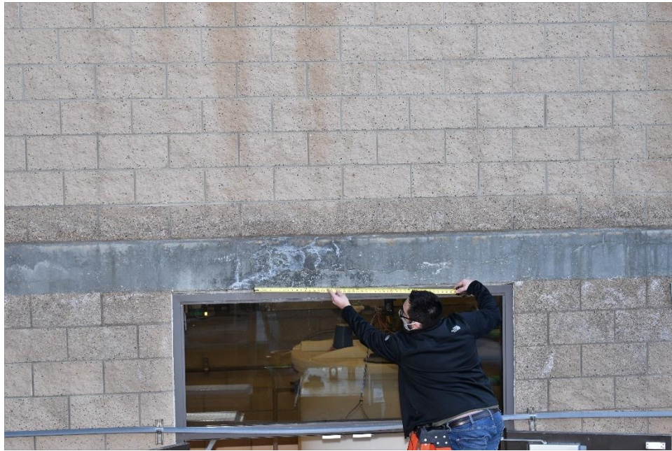
Photograph 15: Damage to Slab Thickened Edge (01/27/2022)
