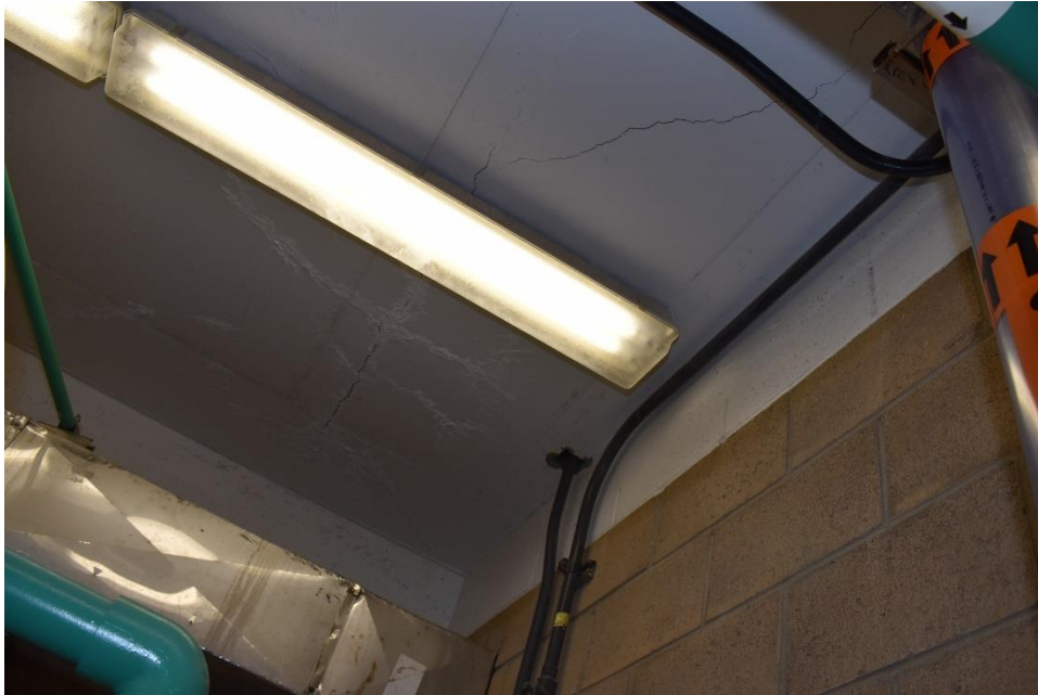
Photograph 13: Cracking in Fluoride Room Ceiling Slab (01/27/2022)
