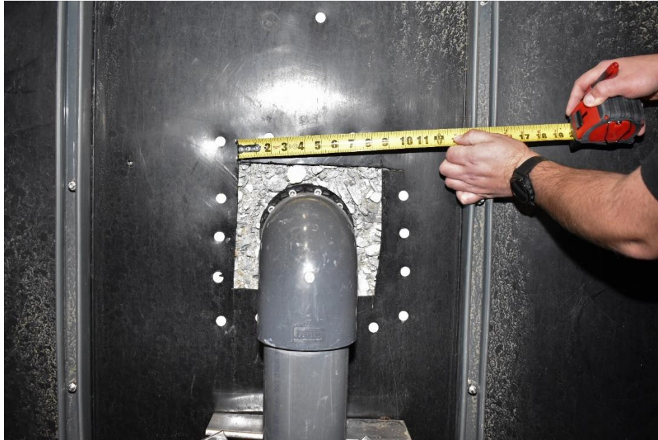
Photograph 1: Concrete at Pipe Penetration on North Wall (01/26/2022)
