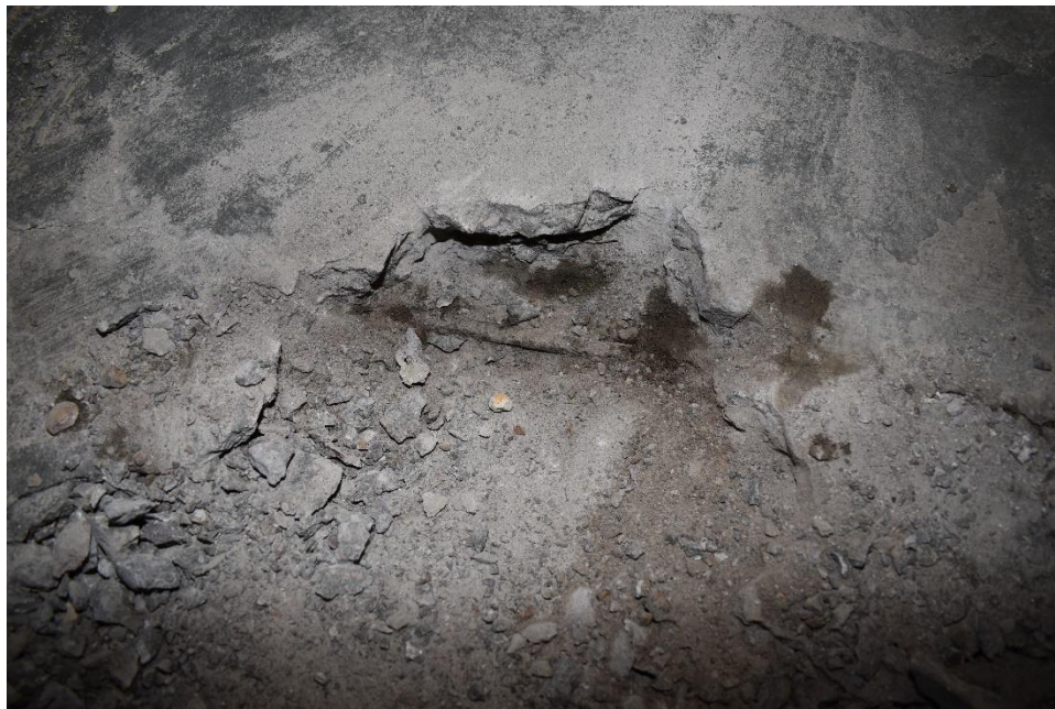
Photograph 21: Exposed reinforcement in Sodium Hypochlorite Room Floor Slab (01/27/2022)
