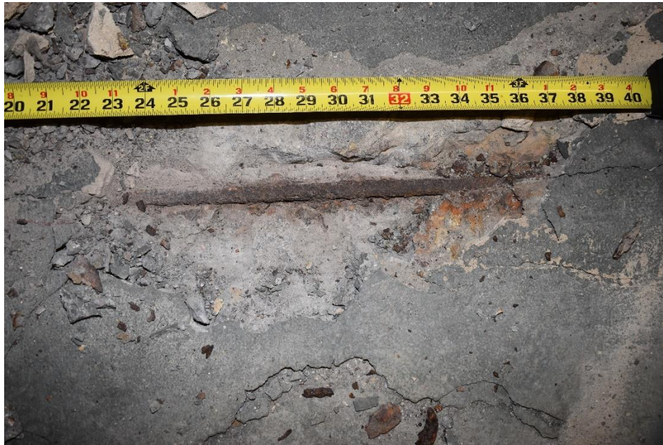
Photograph 20: Exposed reinforcement in Sodium Hypochlorite Room Floor Slab (01/27/2022)
