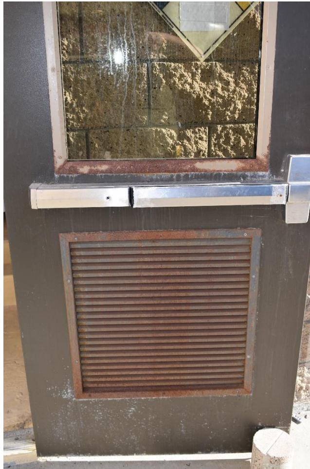
Photograph 19: Corrosion on Door of Fluoride Room (01/26/2022)
