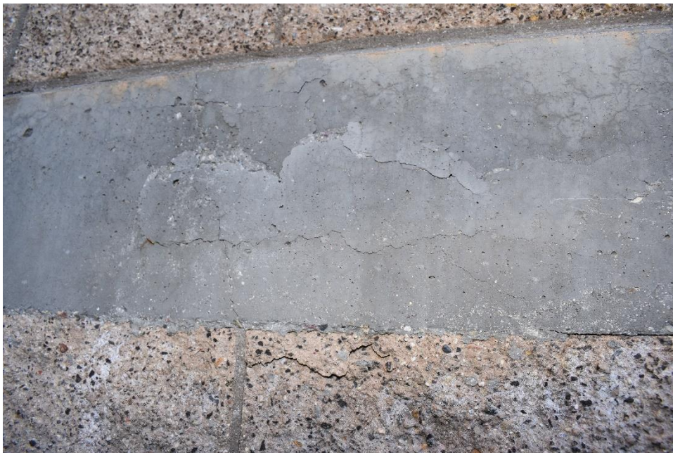
Photograph 14: Cracking and Spalling in Slab Thickened Edge (01/27/2022)
