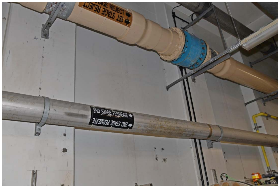
I-32 View of 2 nd stage permeate piping, illustrating random minor corrosion on the piping.
