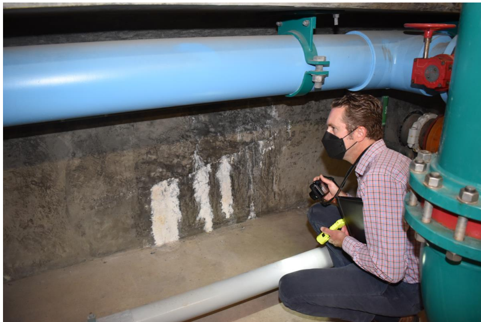
Photograph 8: Crack and Efflorescence in Primary Basins
