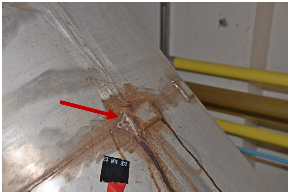
I-19 Same as Photo I-18, except rust scale has been scraped away to examine the substrate.
