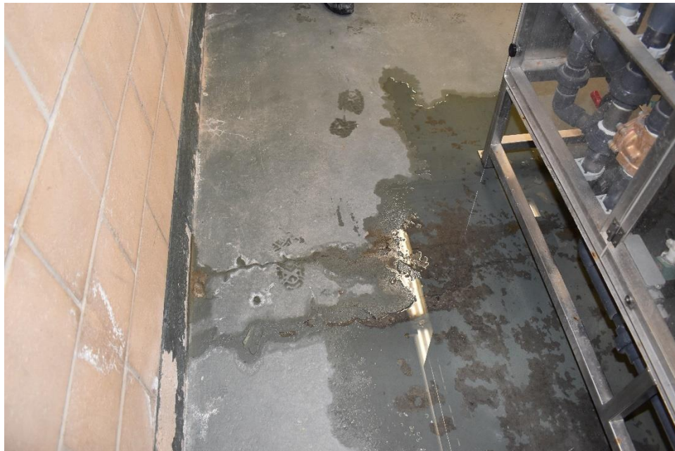
Photograph 10: Leaking from Chlorination System in Sodium Hypochlorite Room (01/26/2022)
