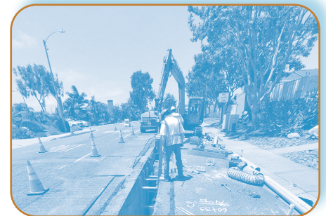
Installing recycled water pipeline
