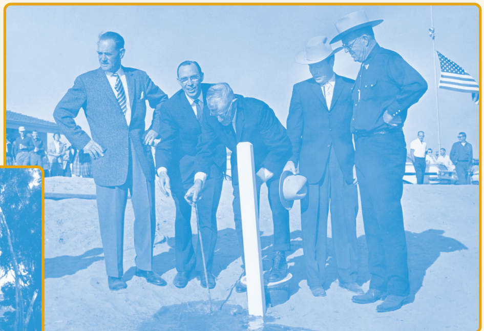
President Wiegand turned on the valve that started the water flowing into newly constructed OMWD pipelines. Board members in 1961 were, left to right, Otto Berk, Howard Golem, Alwin Wiegand, James Wood, and Clarke Thomas.
