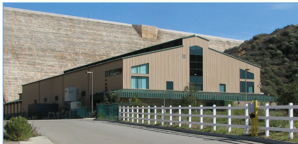
David C. McCollom Water Treatment Plant
