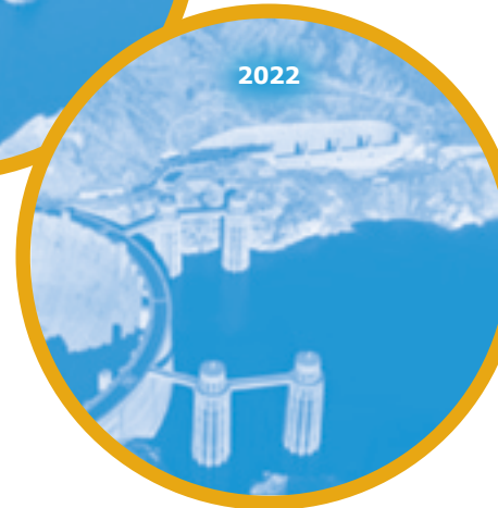
Historic low water levels on Lake Mead have exposed four 338-foot-high intake towers behind the Hoover Dam.
