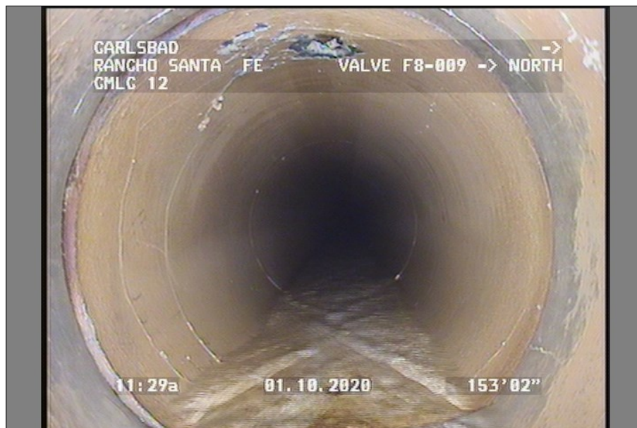
Photo: VALVE F8-009-NORTH-D-153.1533-112744.JPG Crack In Lining
