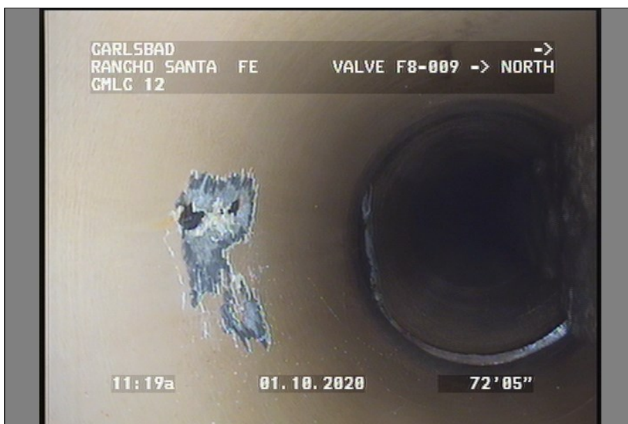
Photo: VALVE F8-009-NORTH-D-72.3885-111720.JPG Crack In Lining
