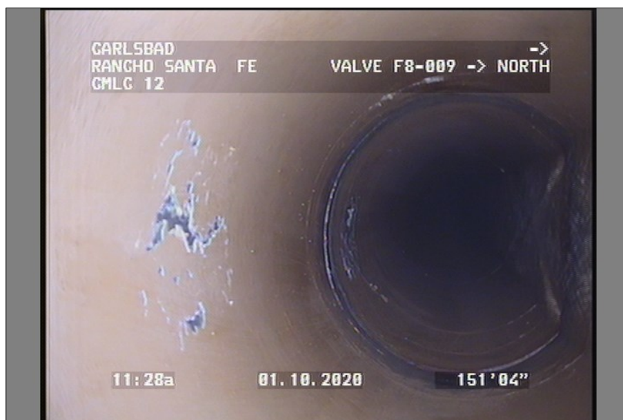
Photo: VALVE F8-009-NORTH-D-151.2919-112648.JPG Crack In Lining
