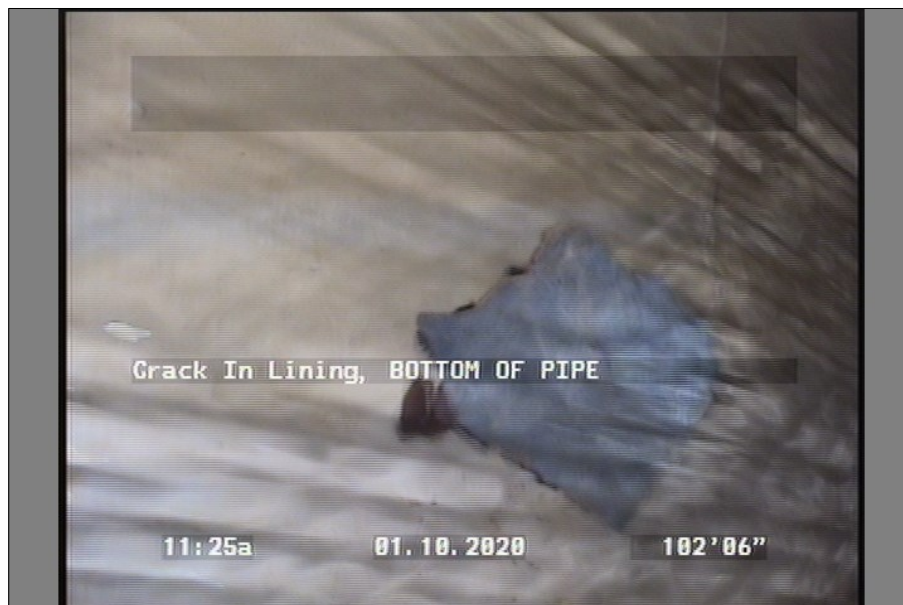
Photo: VALVE F8-009-NORTH-D-102.4814-112341.JPG Crack In Lining
