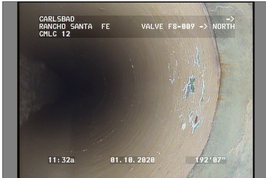
Photo: VALVE F8-009-NORTH-D-192.5533-113020.JPG Crack In Lining
