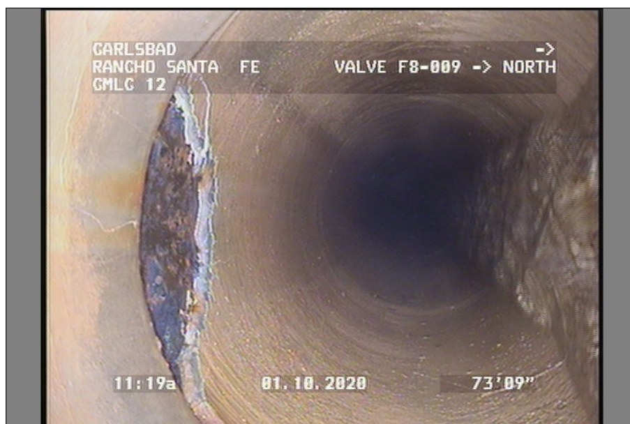
Photo: VALVE F8-009-NORTH-D-73.7328-111816.JPG Crack In Lining
