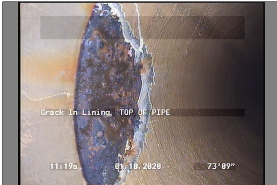
Photo: VALVE F8-009-NORTH-D-73.7328-111808.JPG Crack In Lining
