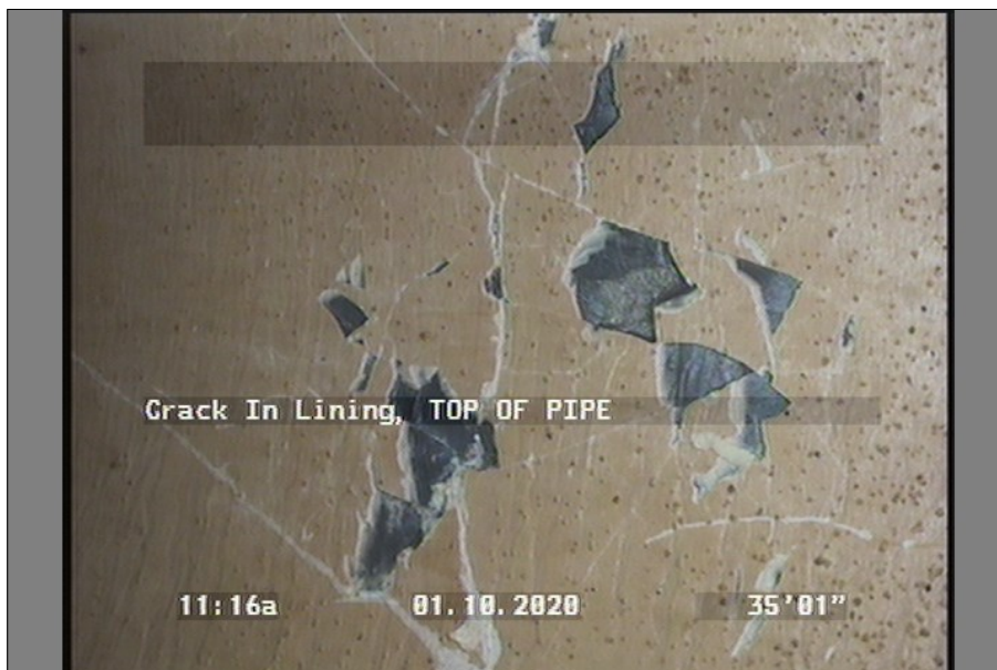
Photo: VALVE F8-009-NORTH-D-35.0567-111451.JPG Crack In Lining
