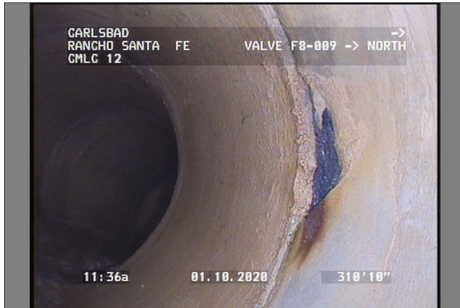
Photo: VALVE F8-009-NORTH-D-310.8567-113430.JPG Crack In Lining
