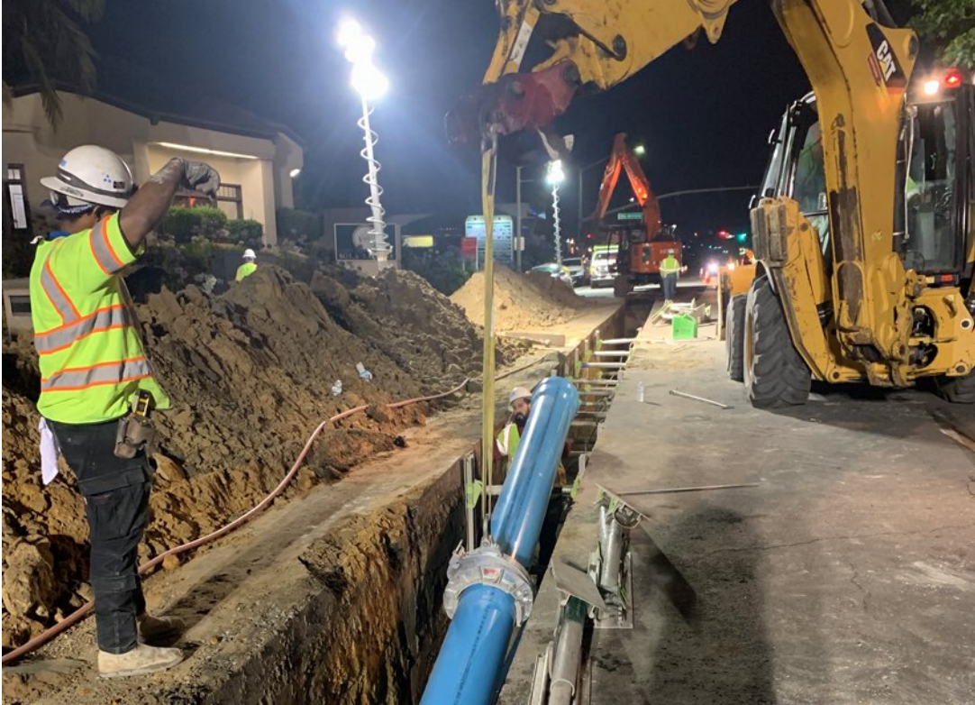
Lowering a section of the new potable water pipe into a trench in El Camino Real. Night work helped minimize the inconvenience to nearby businesses and homes. Photo: Olivenhain Municipal Water District
