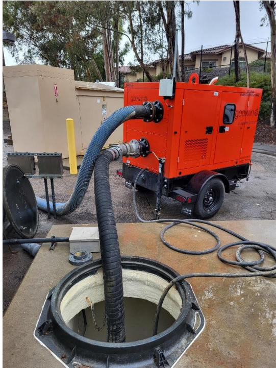
Pumping out of wet well
