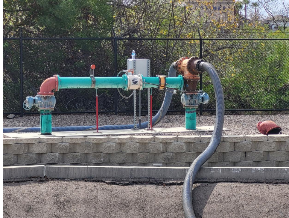
Hoses connected to piping leading to WRF
