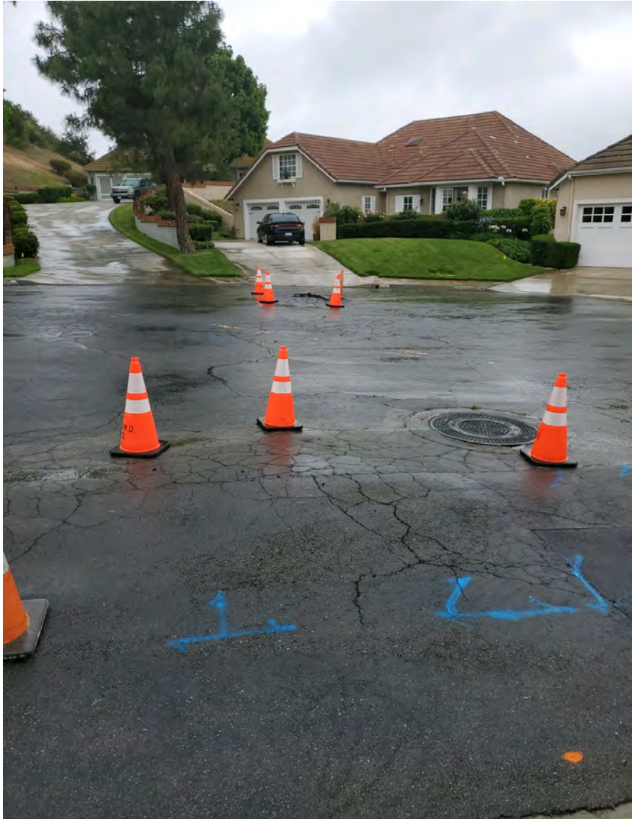
Buckled pavement in the Fox Run Row Cul-de-sac
