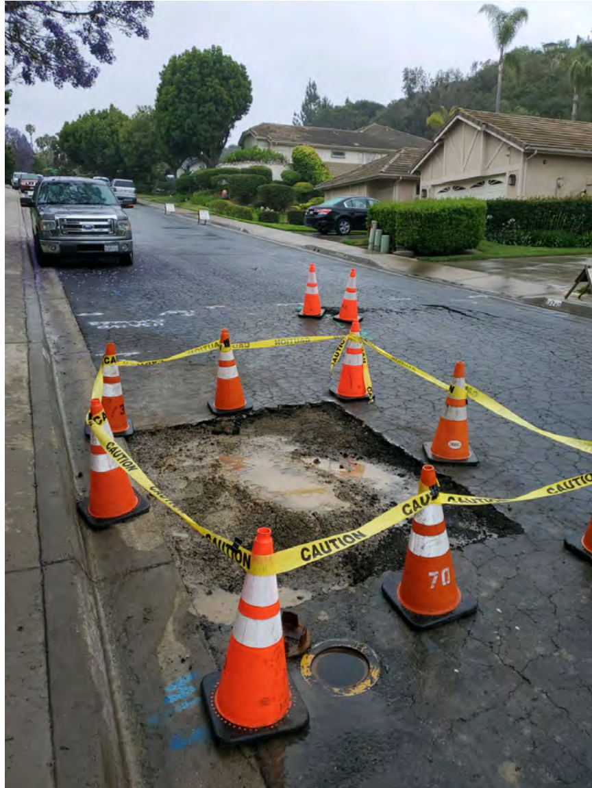
Saturated Pavement on Fox Run Row
