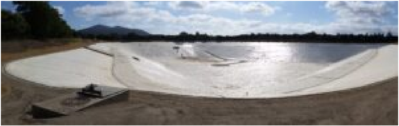
Completed 4S recycled water storage basin with XR-5 Geomembrane.
