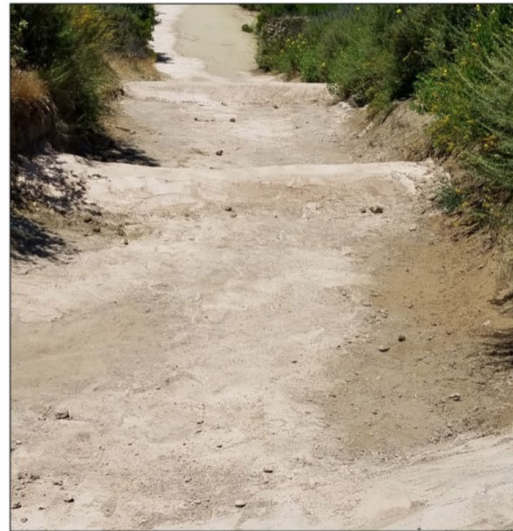
Pipeline stabilization and erosion repair complete with stormwater runoff velocity reduction berms in place.
