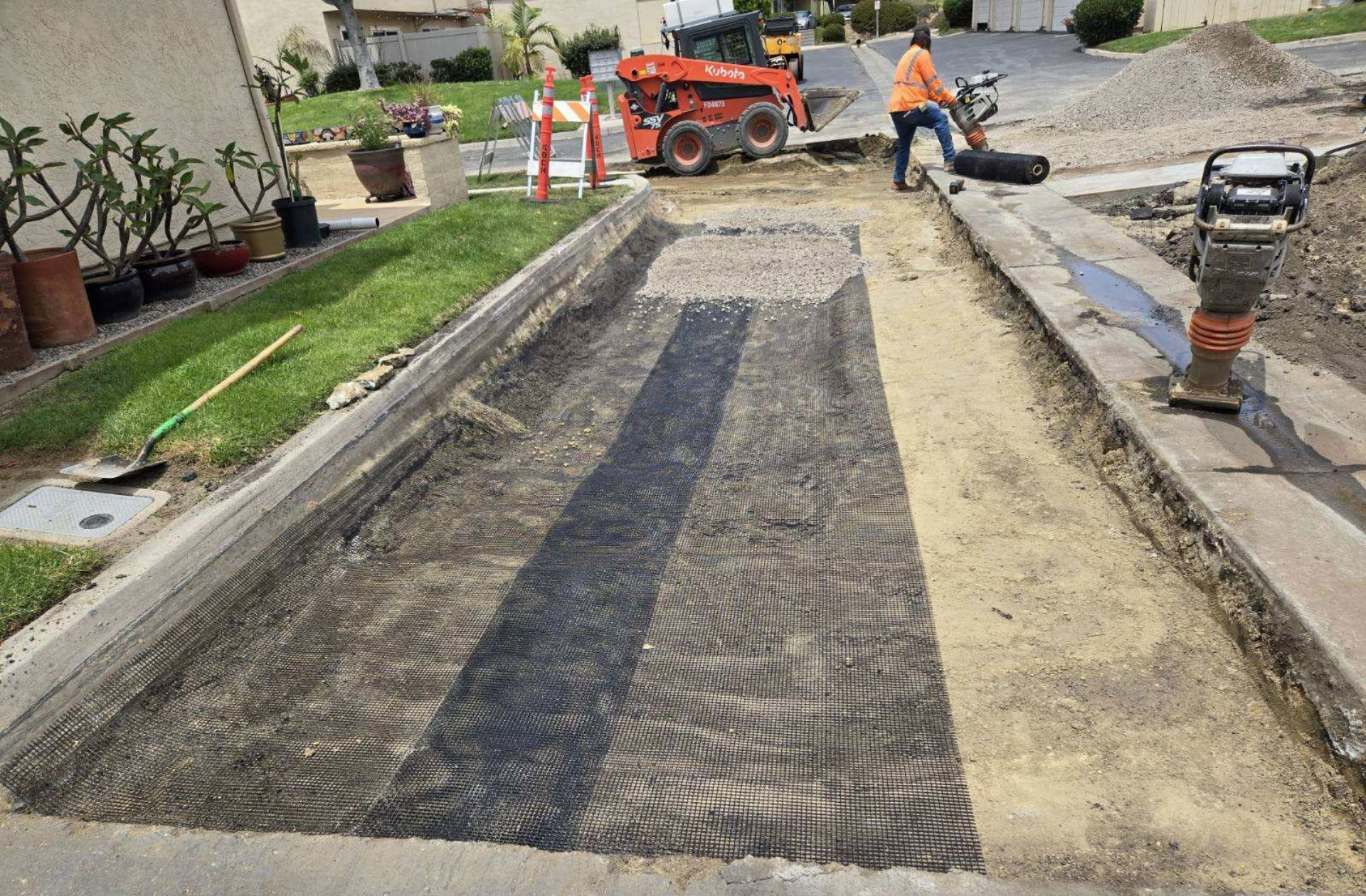
Base Paving With Geo-Grid
