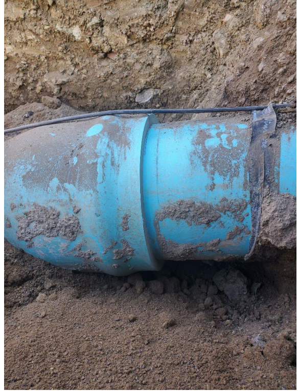
Excavated Sewer Force-Main PVC Pipe (Note dry condition of bedding)
