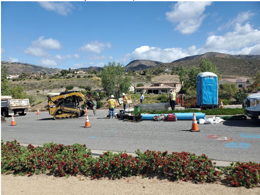
Orion Crews Excavating Sewer Force-Main
