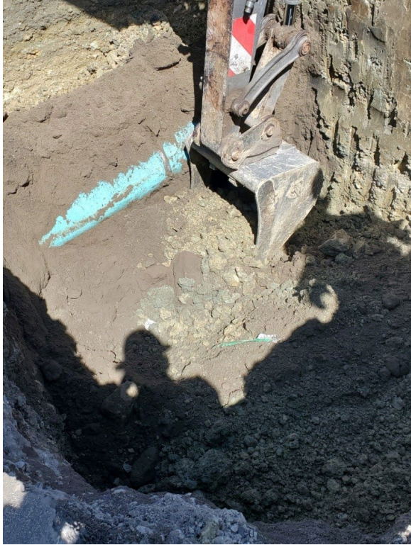
Excavated Sewer Force-Main PVC Pipe (Note dry condition of bedding)
