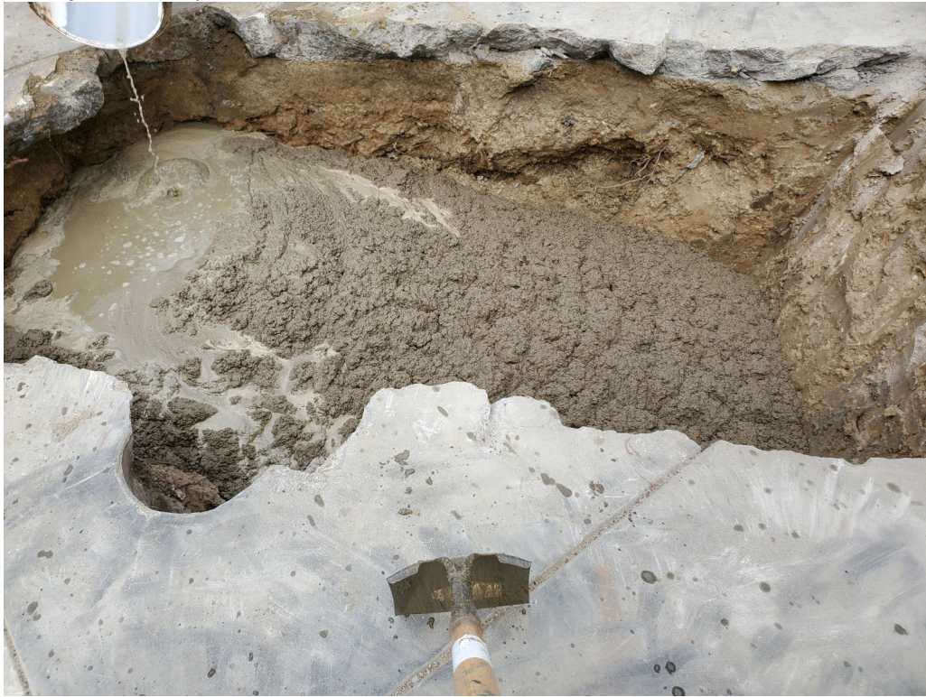
Repair site backfill and compaction
