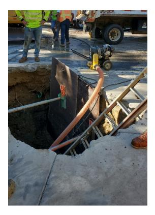
Source of leak: nylon bushing that failed on a 2-inch blow off
