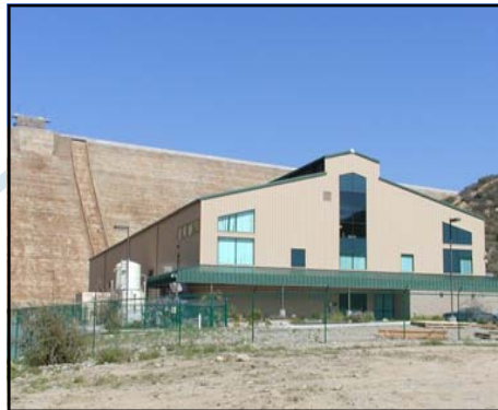
Olivenhain Water Treatment Plant
